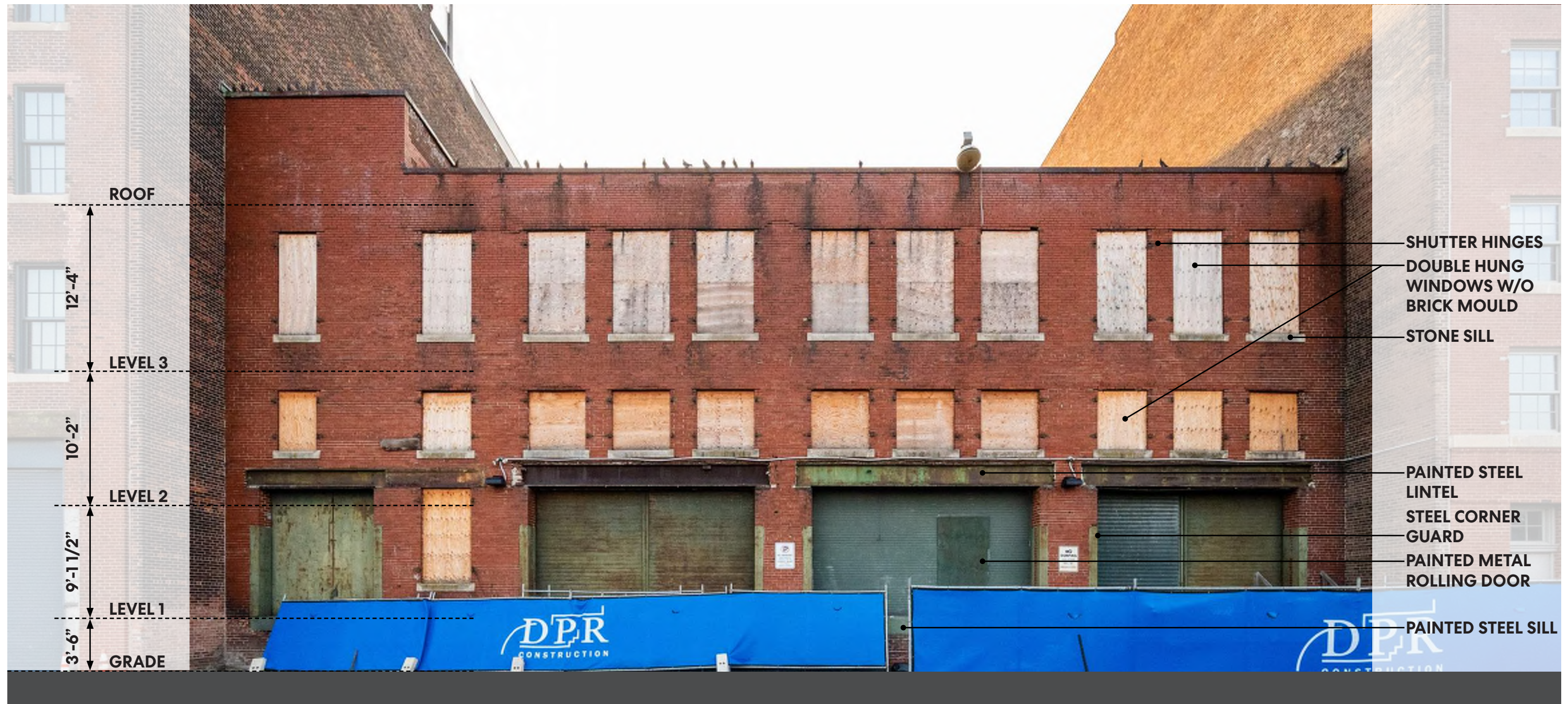
EXISTING FAÇADE - EAST (MEDALLION AVE)
