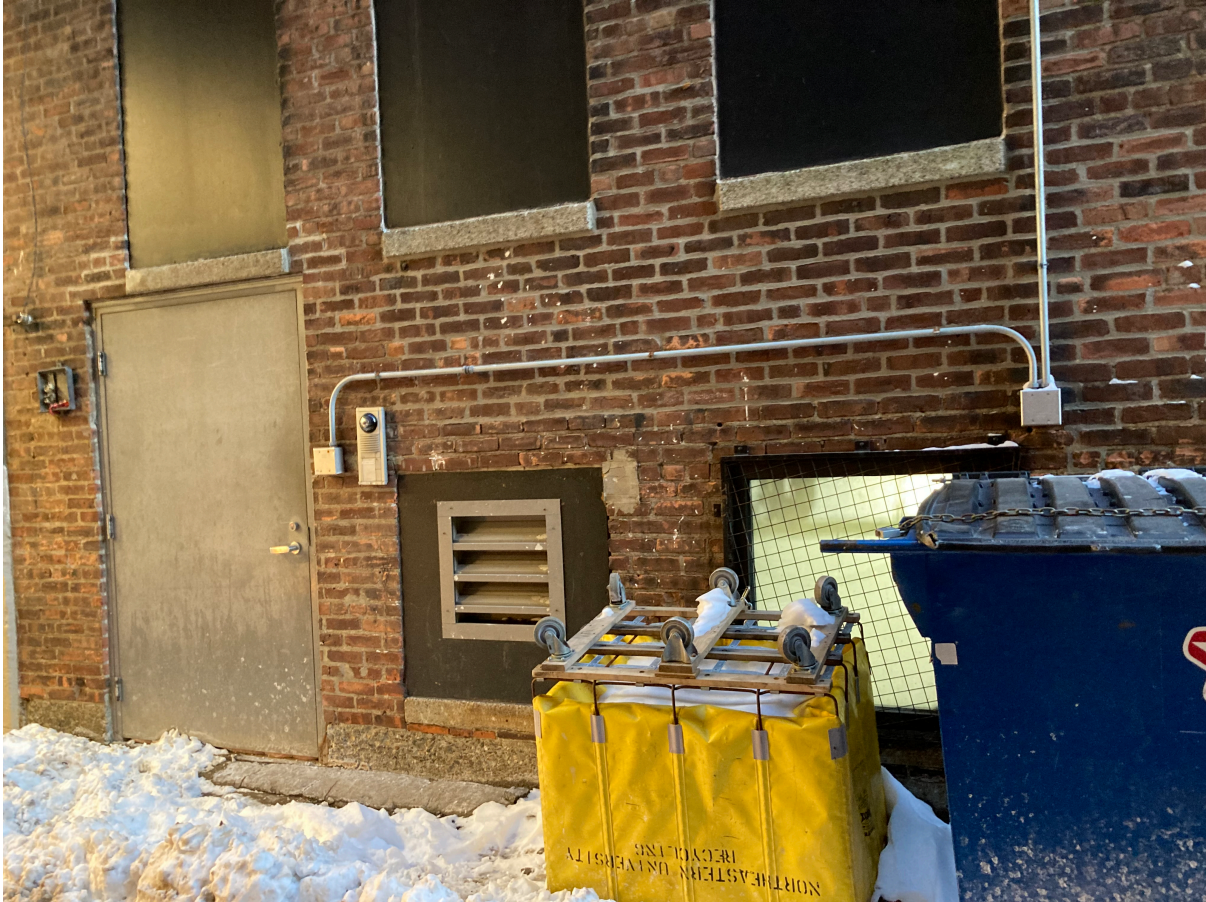
7 - 9 Newbury Street Rear Alley Existing Conditions
