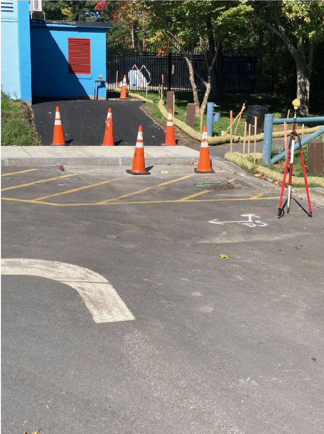
Photo 2 – View of Driveway Binder Layer and Straw Wattles
