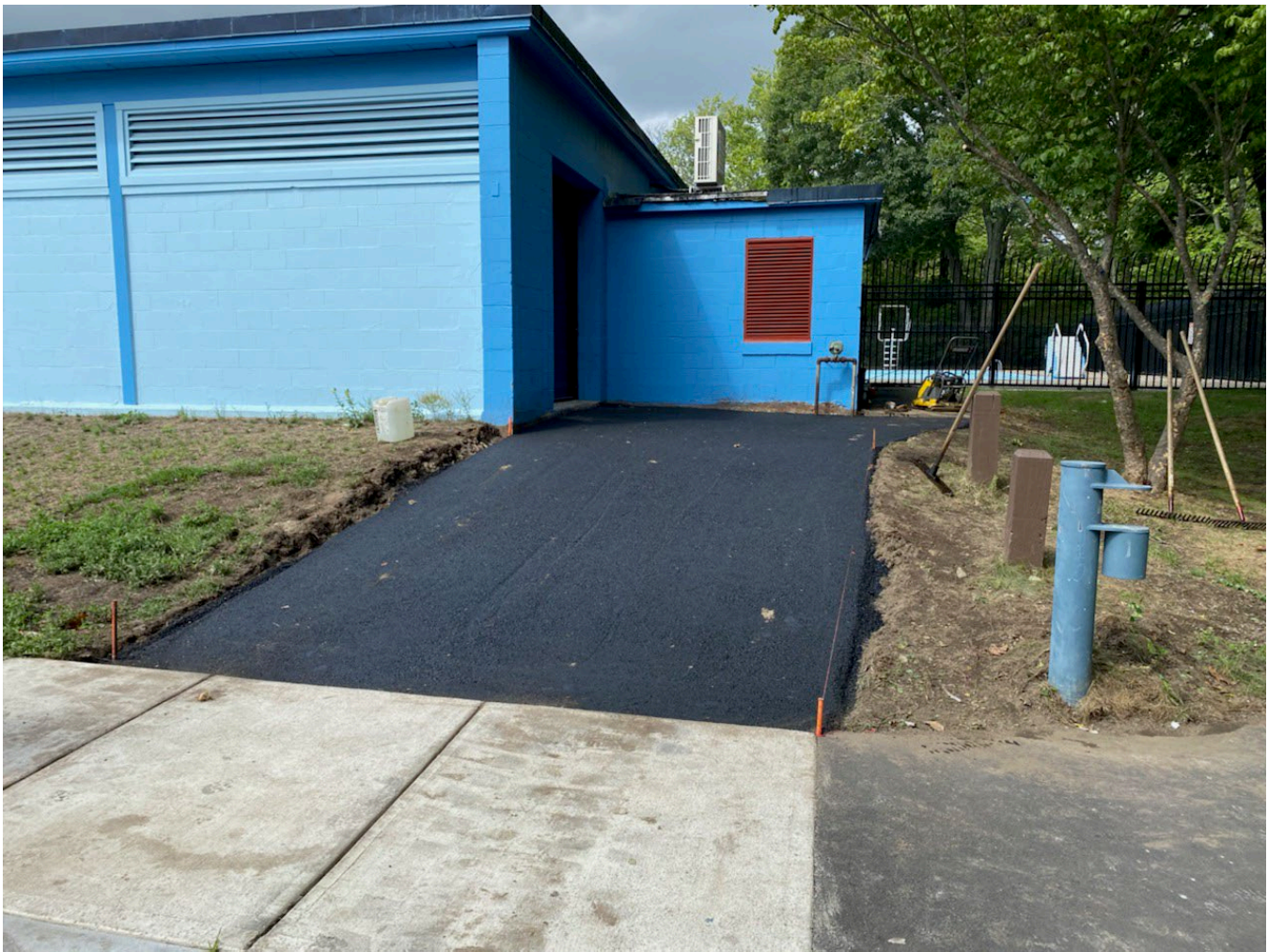
Photo 1 – View of Driveway Binder layer at Bathhouse
