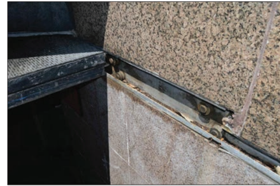
03 ROLL OUT DOOR TRACK SCALE:NTS
