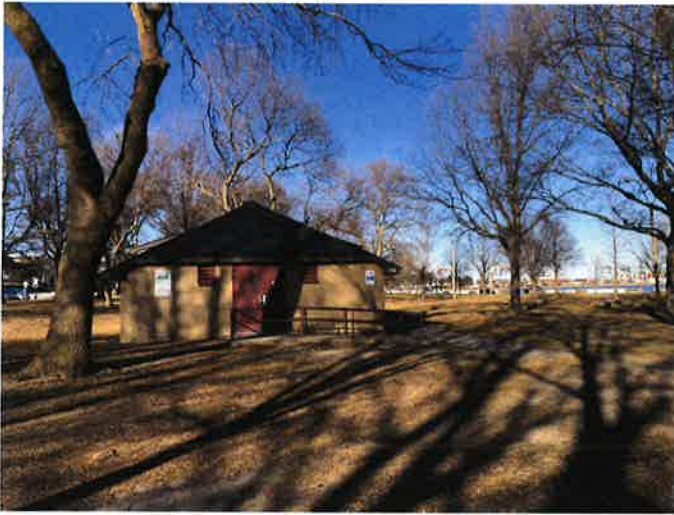
Existing Restroom Facility
