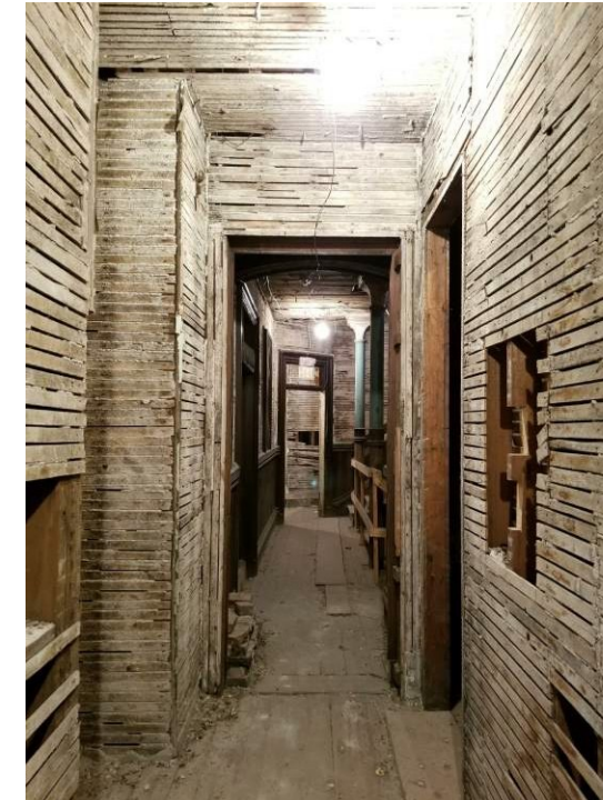
VIEW OF INTERIOR CORRIDOR
