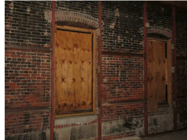
SUPPLEMENTAL BRACING AT EXTERIOR WALL
