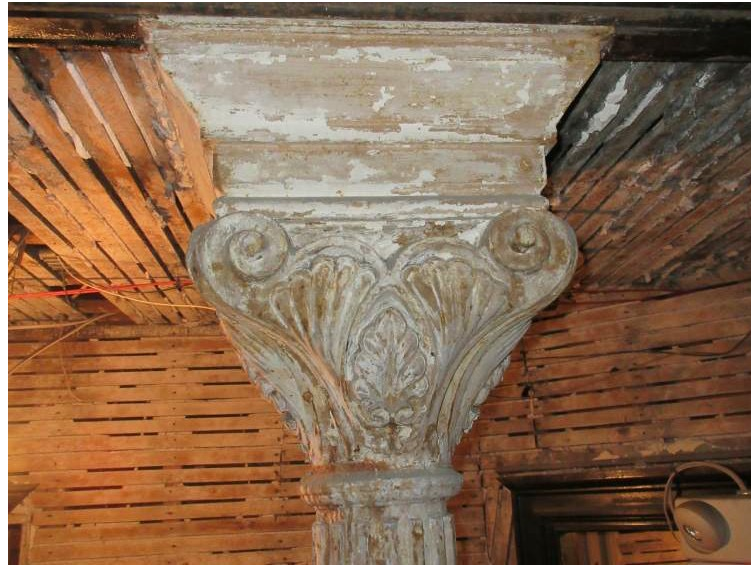
CAST IRON COLUMN CAPITAL
