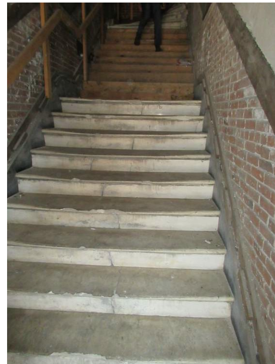
MARBLE ENTRY STAIRS
