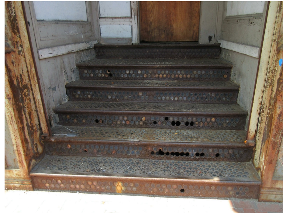
CAST IRON AND PRISM GLASS STAIR MASS AVE
