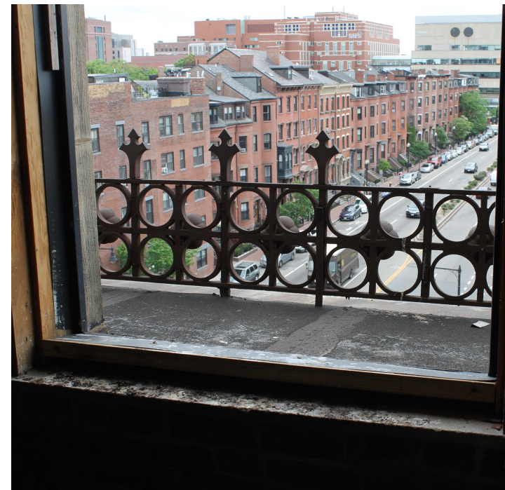
ORIGINALCAST IRON BALCONY RAIL
