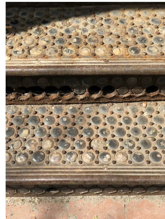
CAST IRON AND PRISM GLASS STAIR DETAIL
