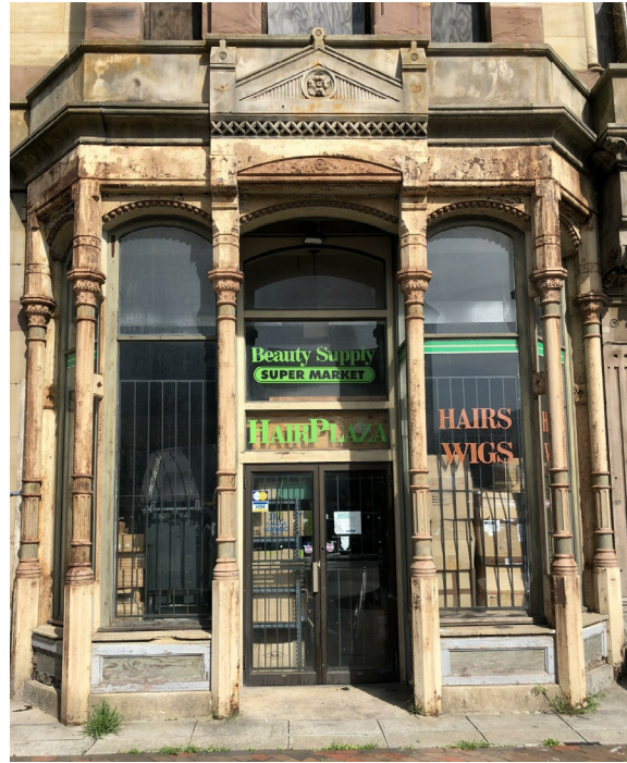
WASHINGTON STREET CAST IRON ENTRANCE
