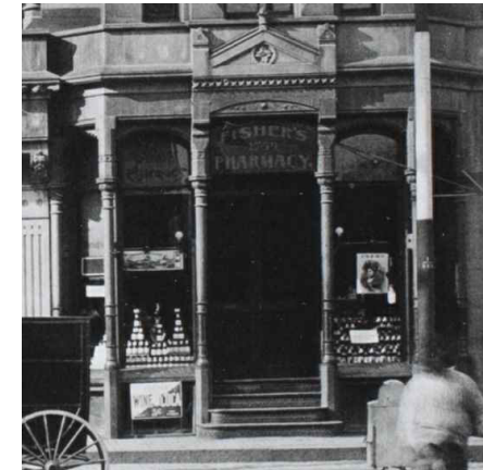
PHOTO 5: 1899 PHOTO SHOWING STORE FRONT WITH CAST IRON STAIRS WITH PRISM LIGHTS AND DOUBLE DOORS
