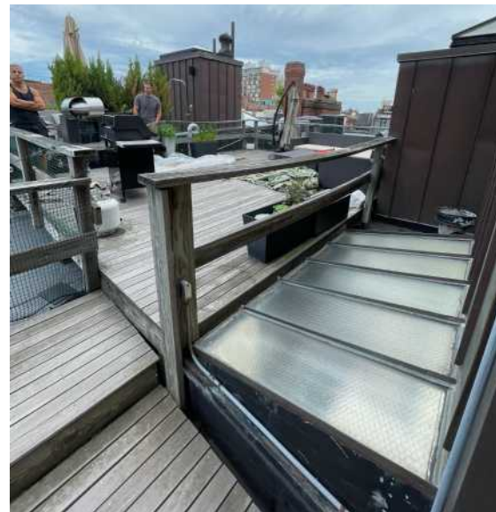
LOOKING NORTH WEST SKYLIGHT & ELEVATOR SHAFT
