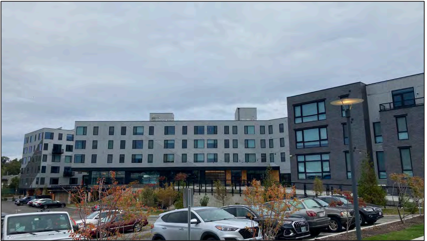
Condition 4: Exterior Building Construction, October 2022
