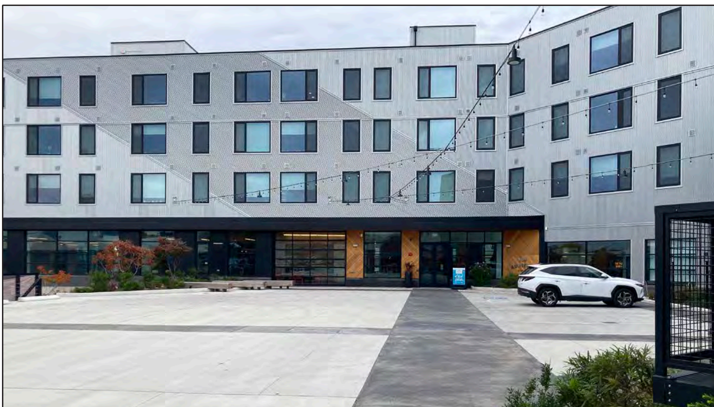
Condition 4: Exterior Building Construction, October 2022
