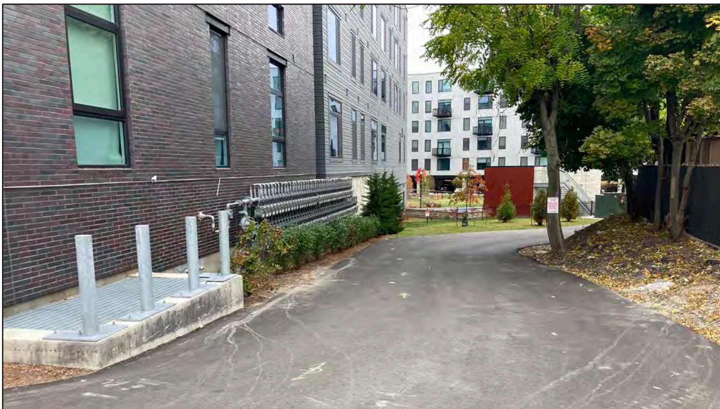
Condition 4: Exterior Building Construction, October 2022
