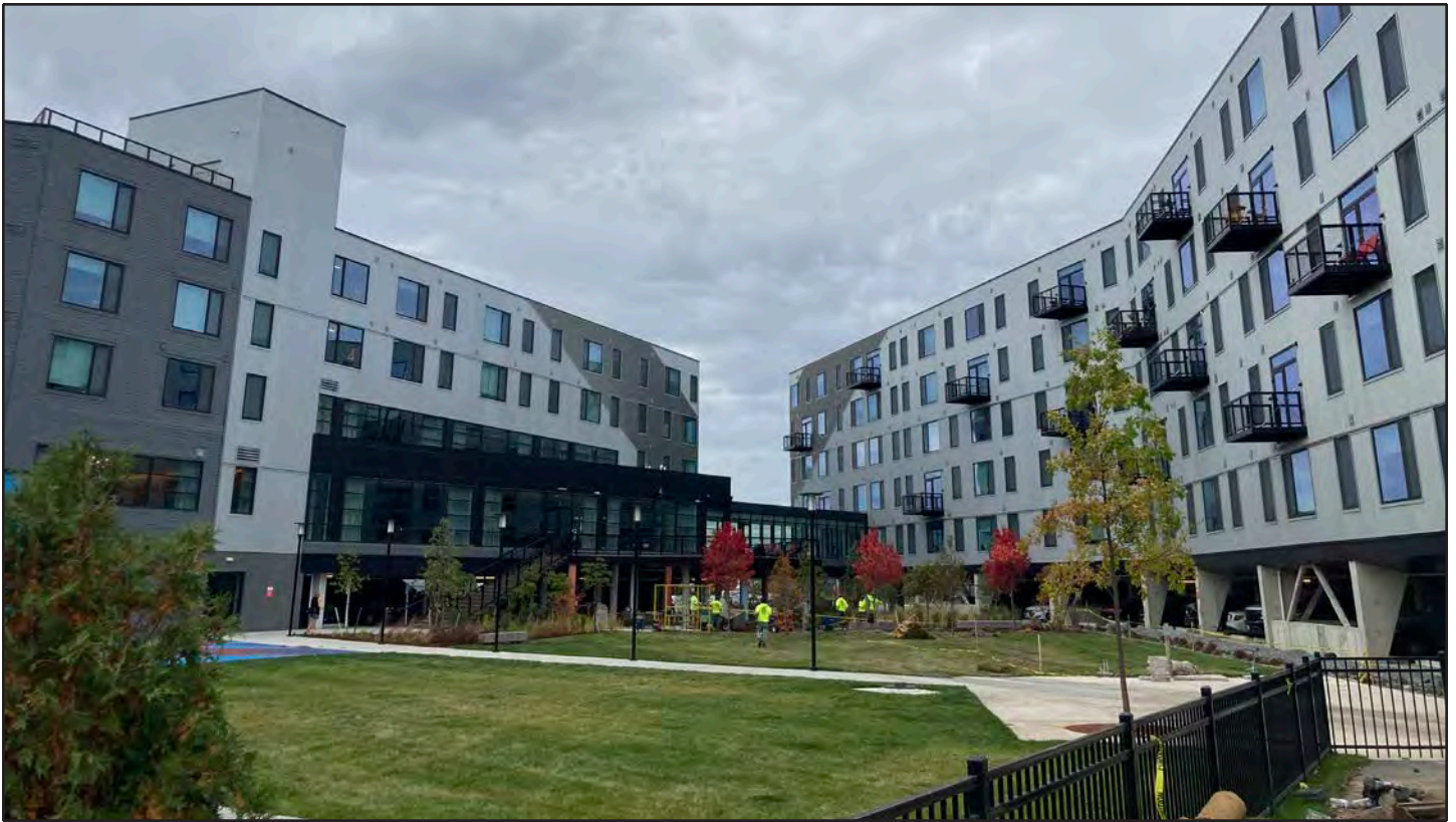
Condition 4: Exterior Building Construction, October 2022
