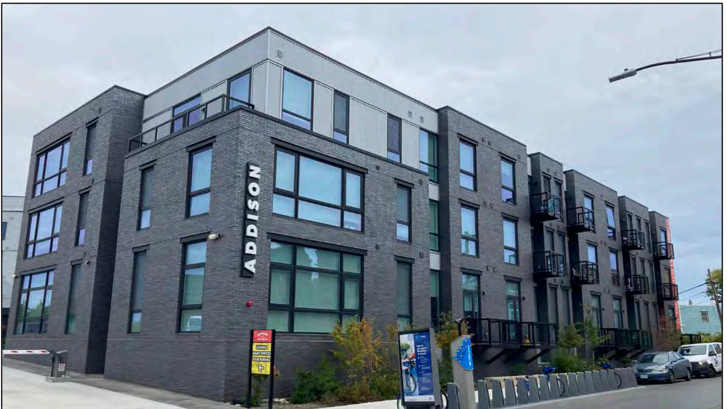
Condition 4: Exterior Building Construction, October 2022
