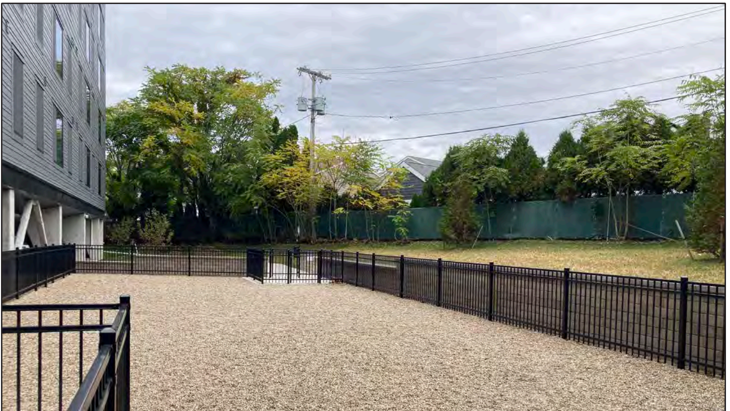
Condition 4: Exterior Building Construction, October 2022
