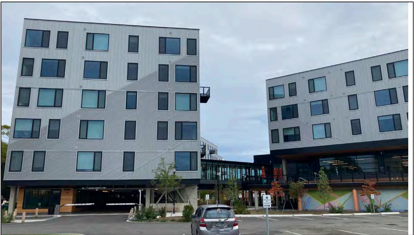
Condition 4: Exterior Building Construction, October 2022
