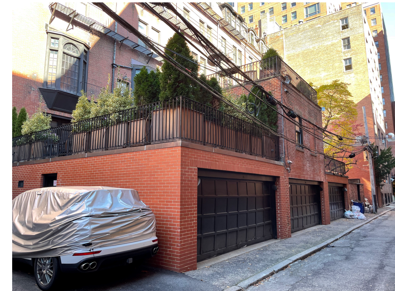
PRECEDENCE: RAILING WITH PLANTERS BEYOND BLACK PAINTED WOOD GARAGE DOORS
