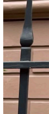
REPLICATE TOP PICKET @ THICKNESS OF VERTICAL POSTS.
