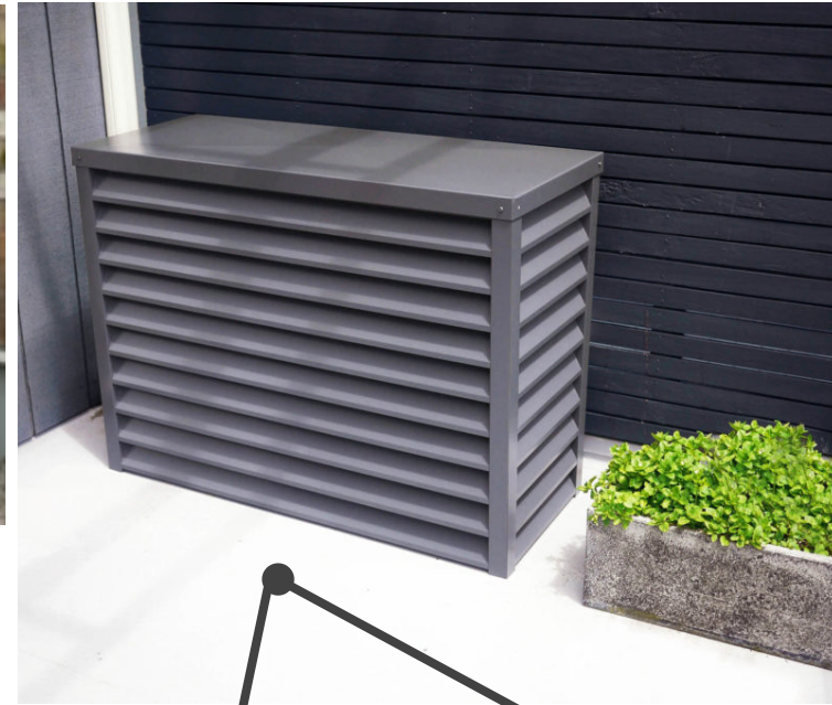
CONCEAL CONDENSERS WITH DARK SURROUND TO MATCH ROOF OR PAINT TO MATCH ROOF AND BRICK
