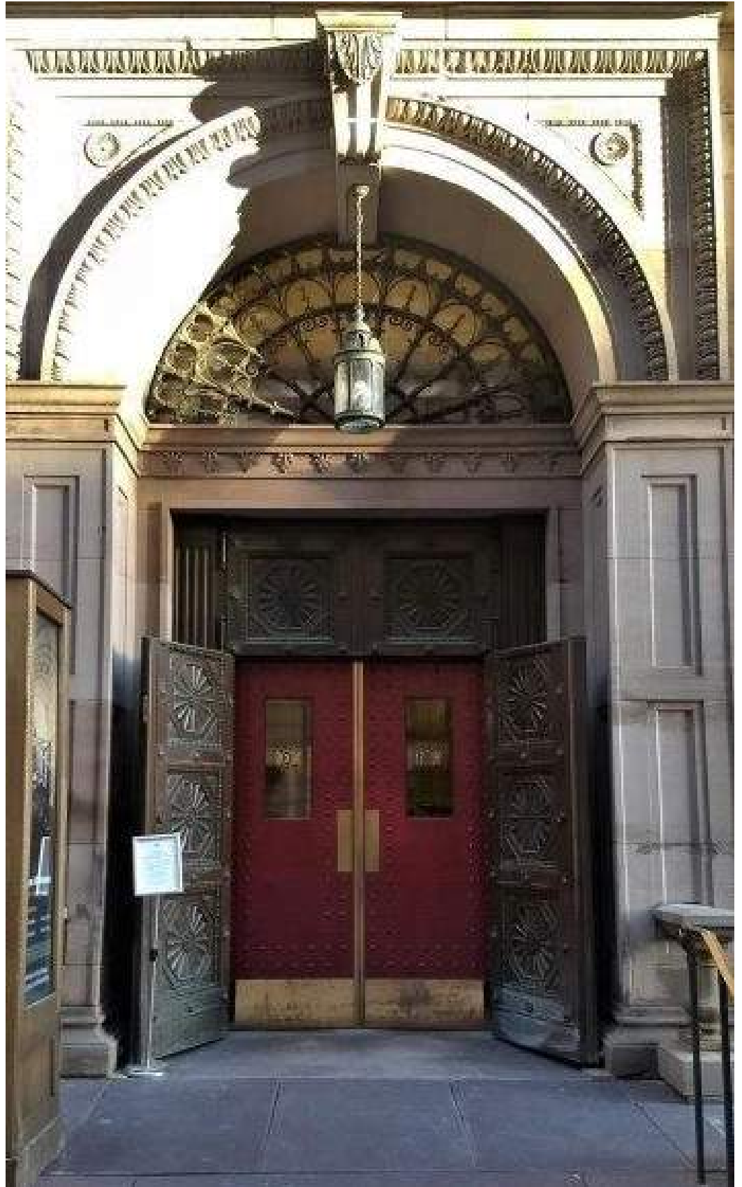
Existing Conditions - Exterior View of Entry Doors
