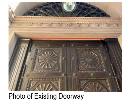
Upper run of Type LB surface mounts to ledge and uplights upper entry facade. Locate remote power supply in a concealed, dry, and accessible location. Lower run of Type LB surface mounts as shown by the solid red line to downlight doorway. Locate remote power supply in a concealed, dry, and accessible location.
