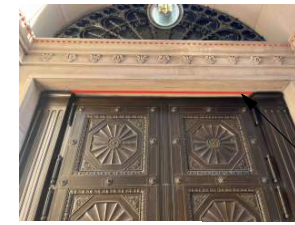
Photo of Existing Doorway
