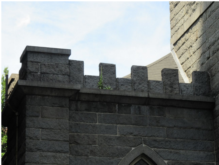
5. 35 Bowdoin Street, roof detail, view northwest
