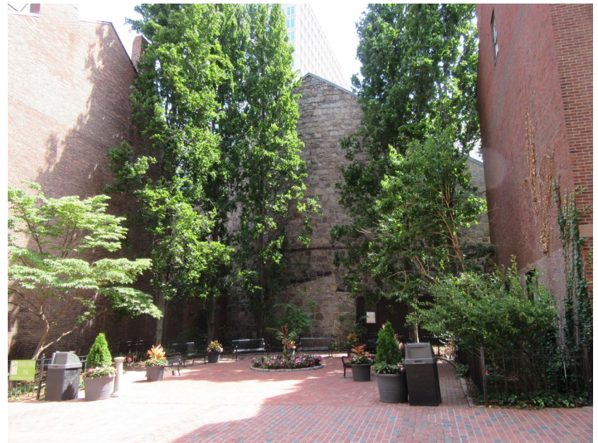
6. 35 Bowdoin Street, west elevation, view northeast from Temple Street
