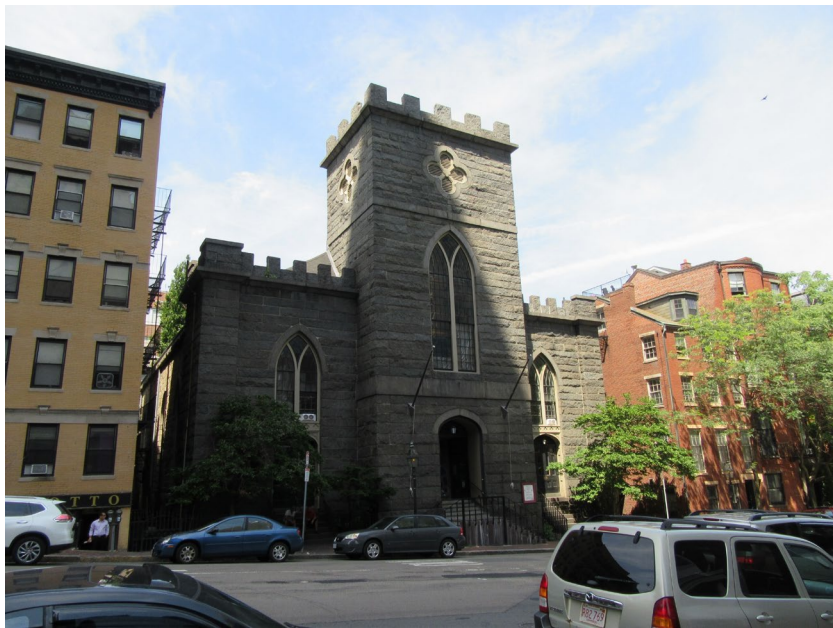
1. 35 Bowdoin Street, front (east) elevation, view northwest
