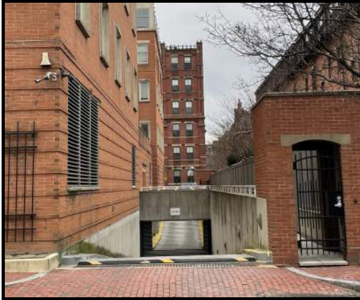
EXISTING GARAGE ENTRANCE RAMP
