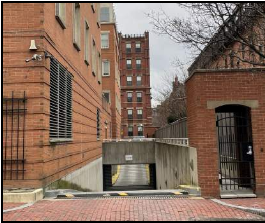
EXISTING GARAGE ENTRANCE RAMP
