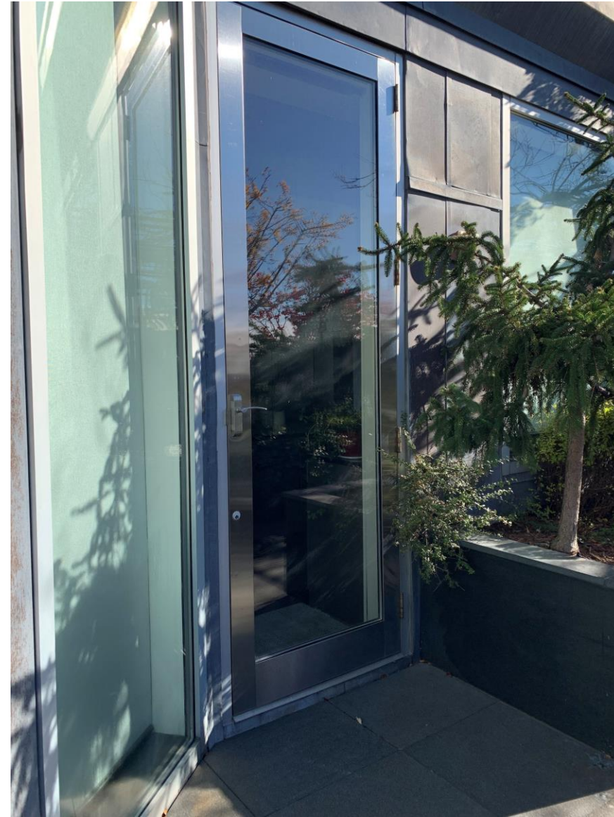
Existing lower floor outswing door
