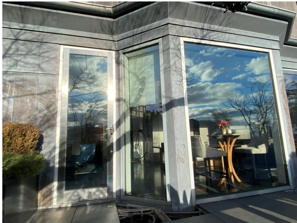
Existing lower floor outswing door and fixed windows
