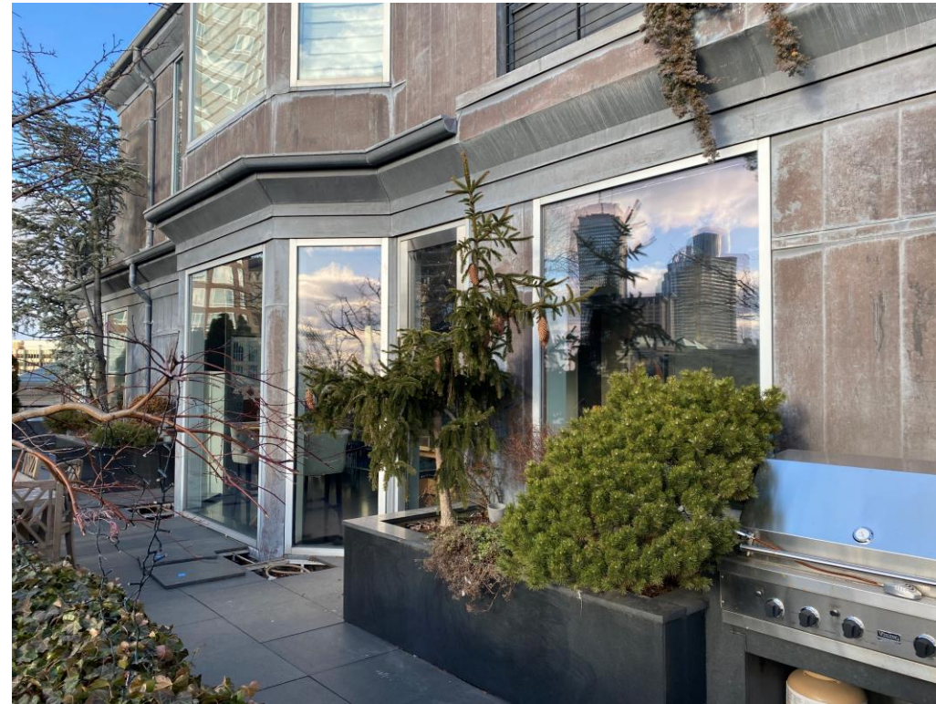
Existing lower floor fixed windows
