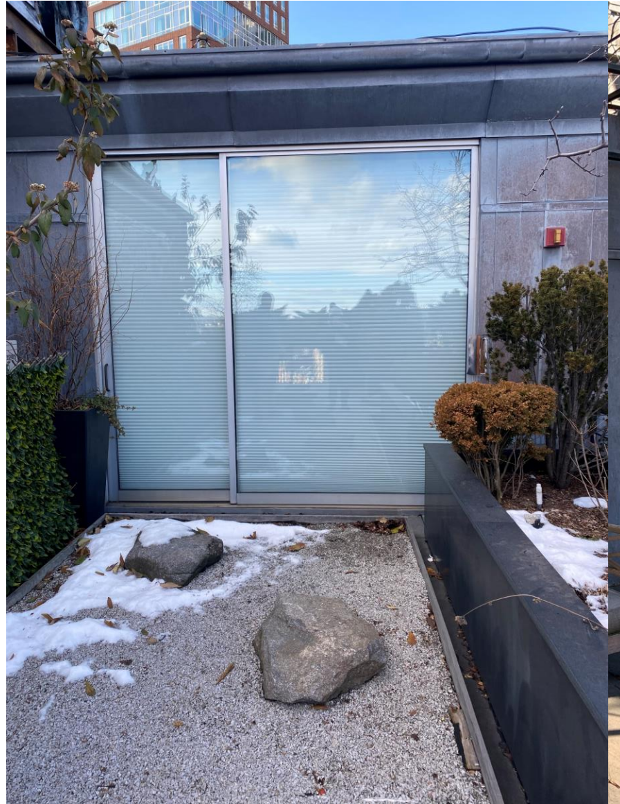
Existing upper floor fixed window and slider door
