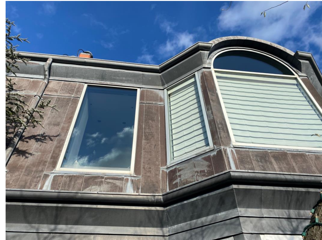
Existing upper floor fixed windows
