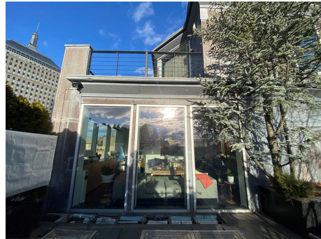
Existing lower floor fixed windows
