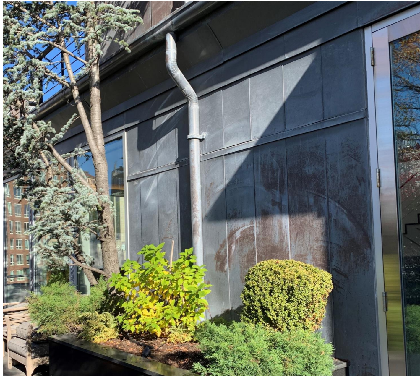
Existing patinaed lead-coated copper cladding
