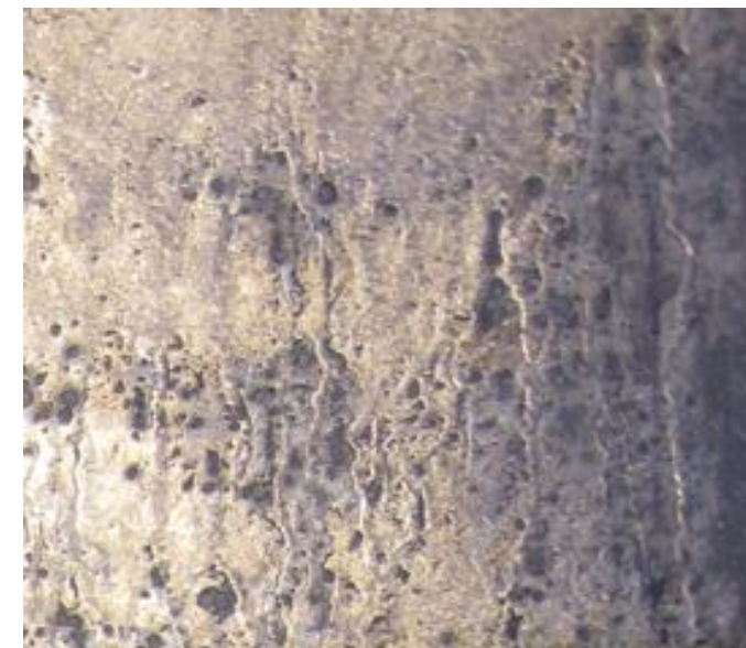
New lead-coated copper cladding appearance
