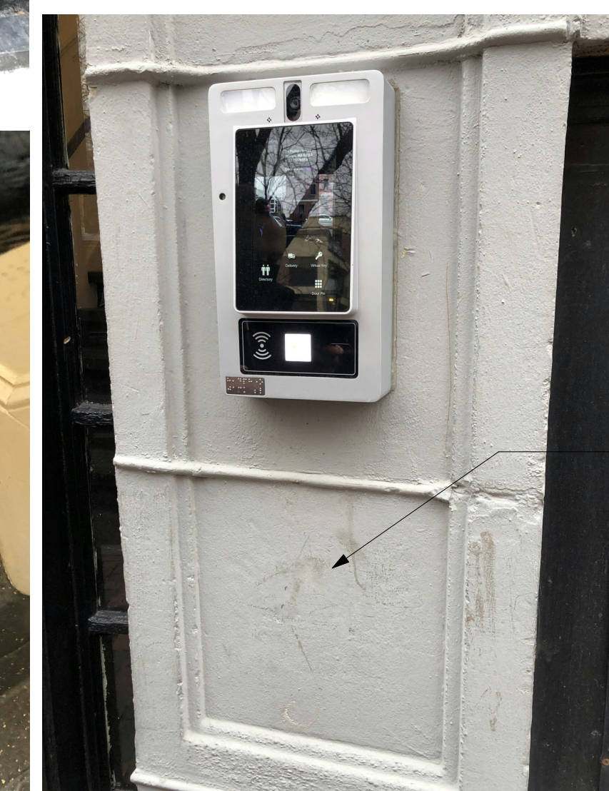
REPAIR & PATCH DAMAGED FACADE BELOW BUTTERFLY
