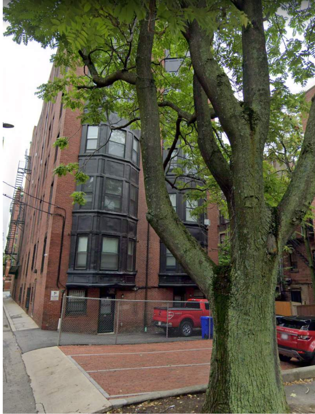
PUBLIC ALLEY 908 LOOKING EAST
