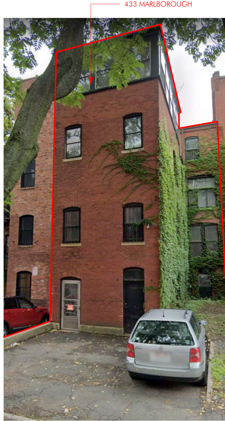
433 MARLBOROUGH ST REAR FACADE
