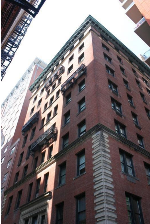
Figure 16. Parker House Annex; upper part of front façade (Bosworth Street). July 2020.
