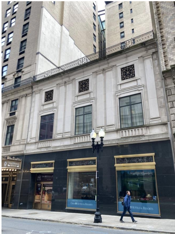
Figure 10. Tremont Street façade; south appendage. October 2021.
