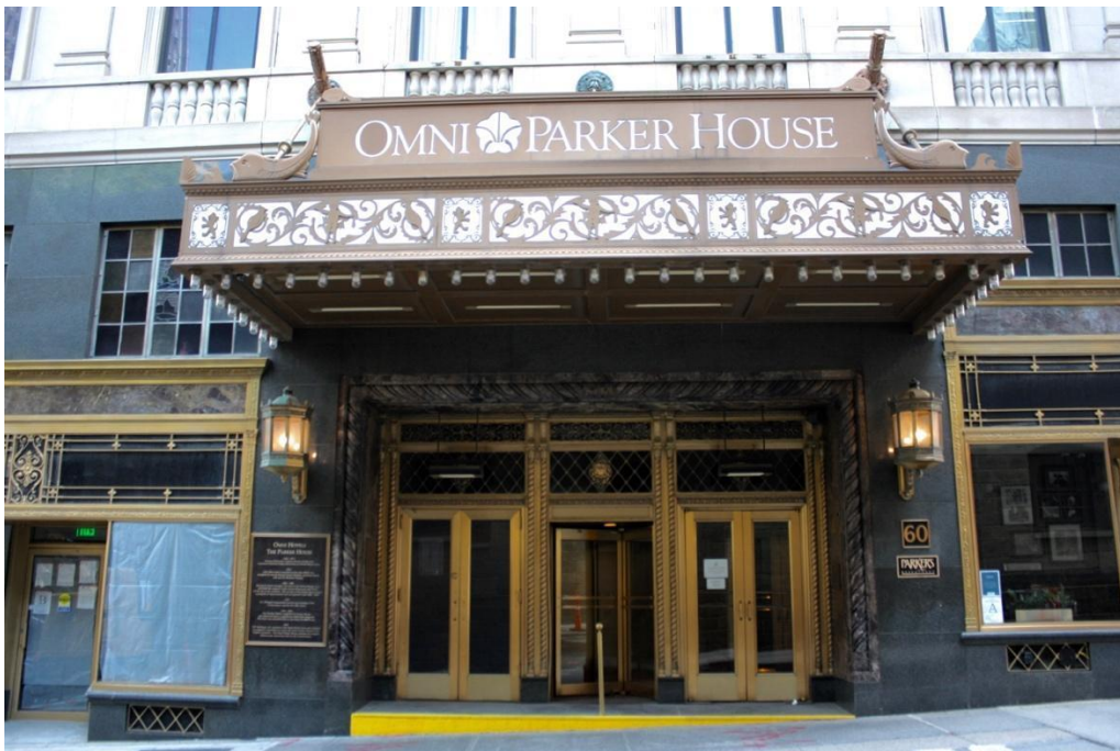
Figure 8. School Street elevation; detail of main entrance. July 2020.
