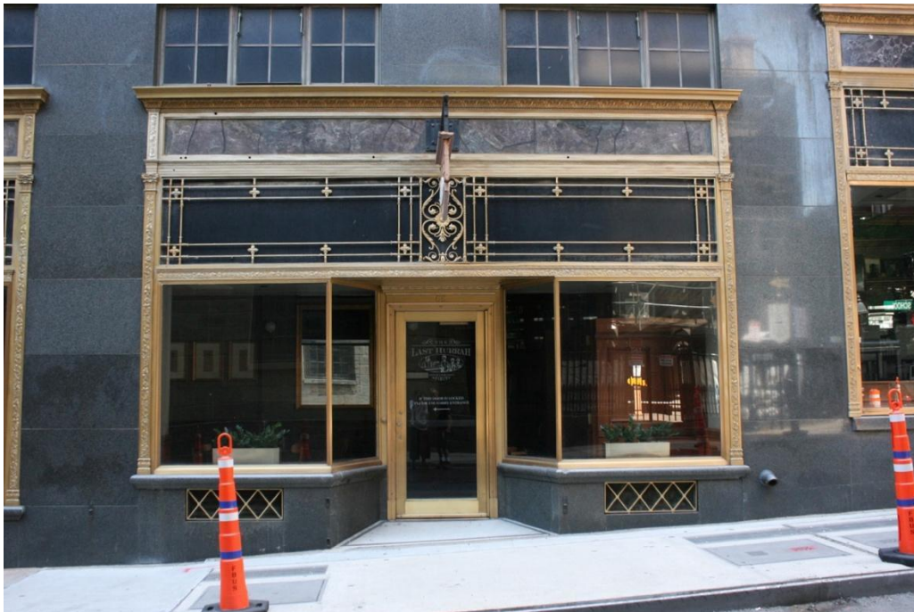
Figure 6. School Street façade, typical storefront. July 2020.
