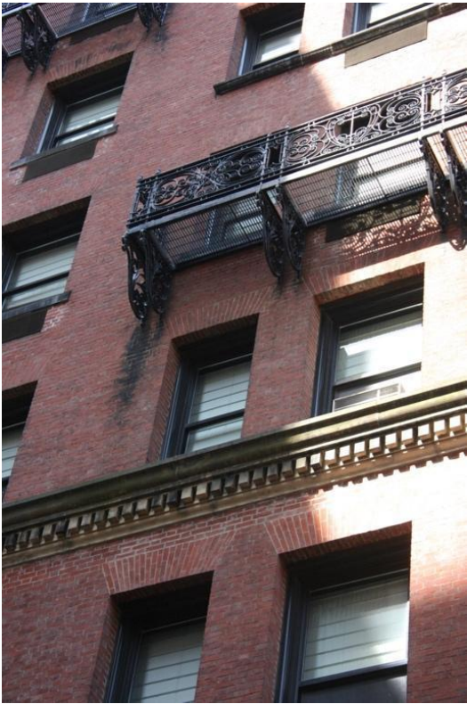
Figure 20. Parker House Annex; detail of façade. July 2020.
