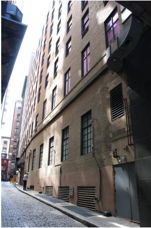
Figure 13. Chapman Place elevation, from School Street. July 2020.
