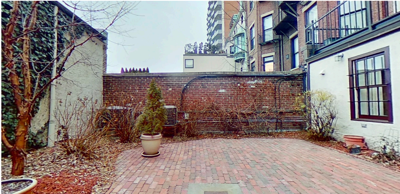
G. WEST COURTYARD FACADE
