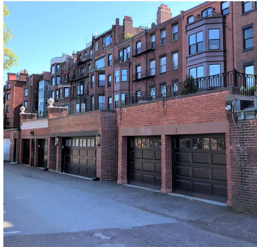
472, 474, 476 BEACON STREET NEW GARAGES WITH ROOF DECKS AND CONNECTING BRIDGES
