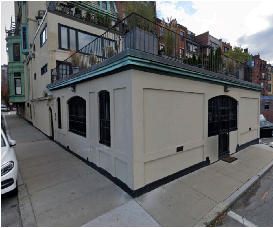
334 BEACON STREET REAR ROOF DECK
