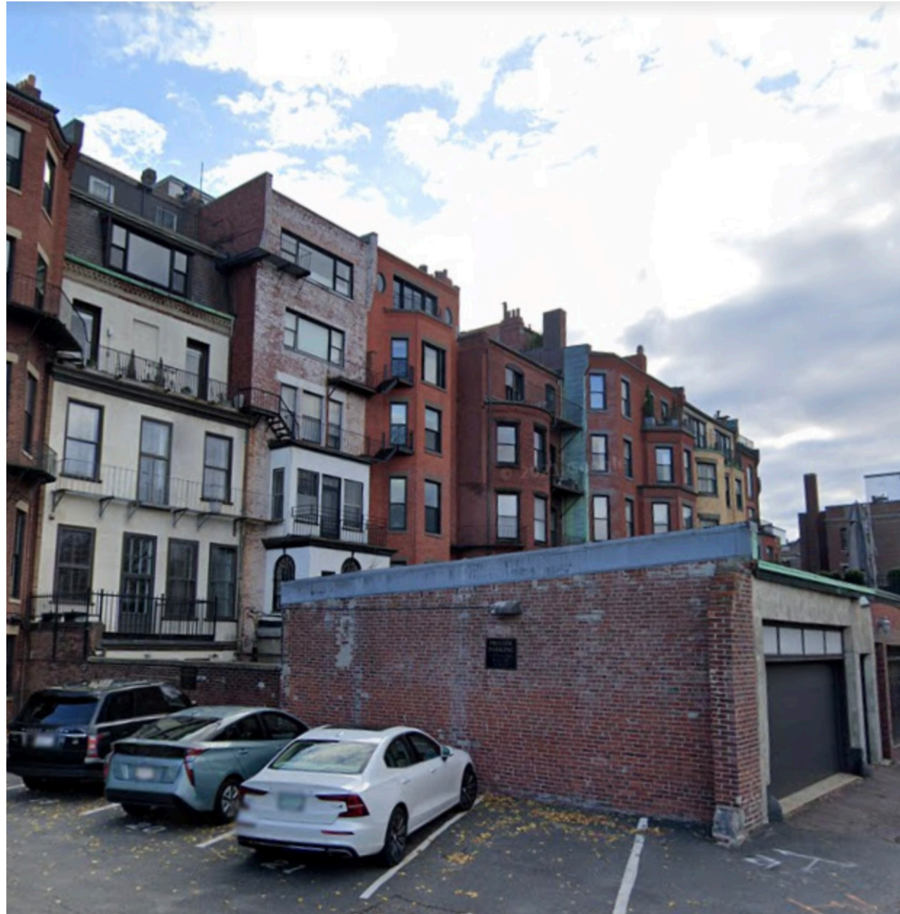
C. EAST GARAGE FACADE - VISIBILTY FROM BACK STREET
