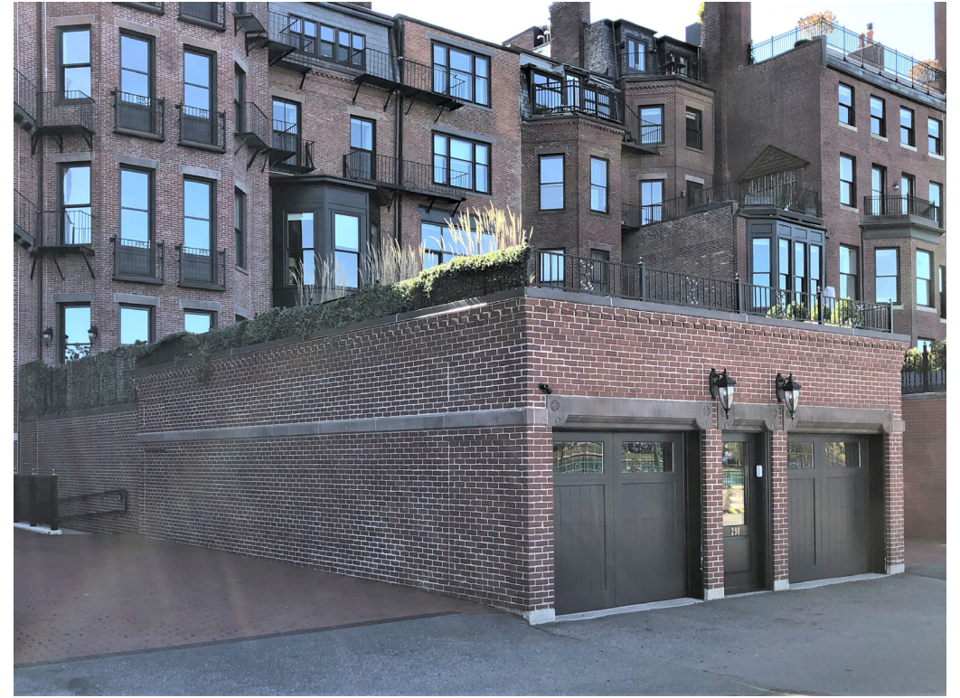
298 BEACON STREET NEW GARAGE WITH ROOF DECK AND CONNECTING BRIDGE
