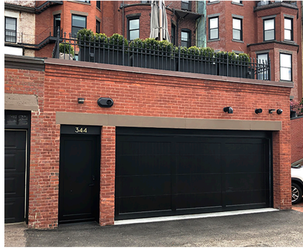
344 BEACON STREET REAR GARAGE WITH ROOF DECK
