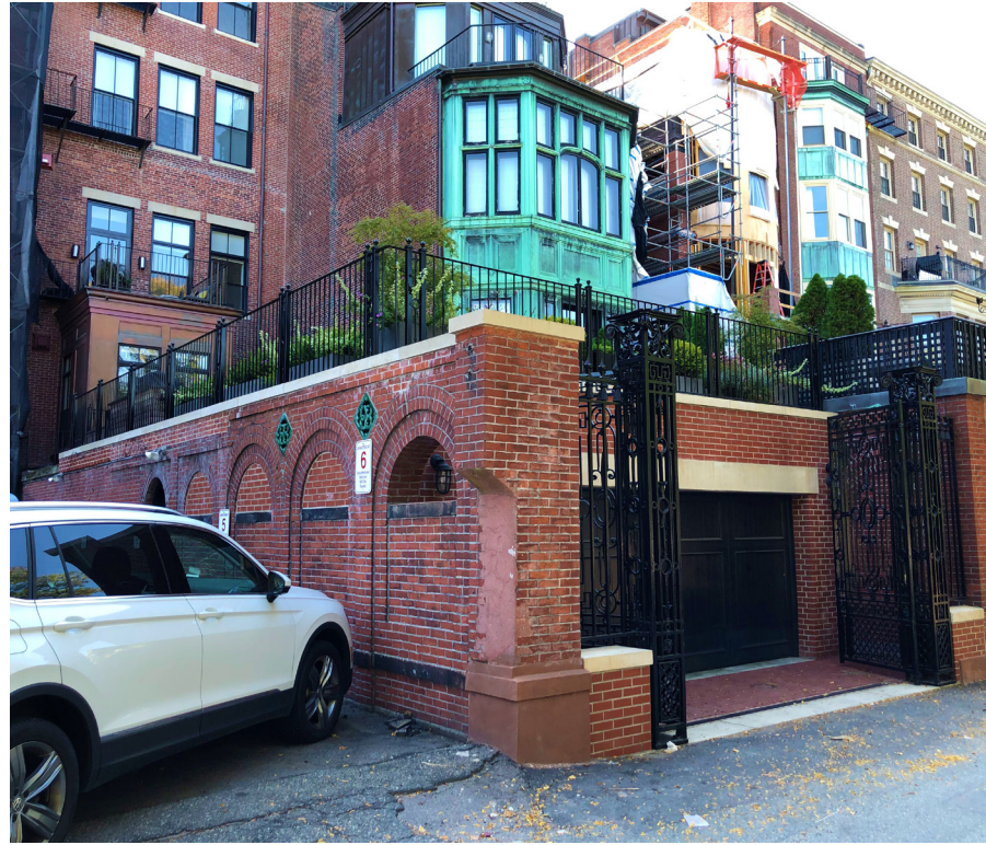
142 BEACON STREET NEW GARAGE WITH ROOF DECK AND CONNECTING BRIDGE
