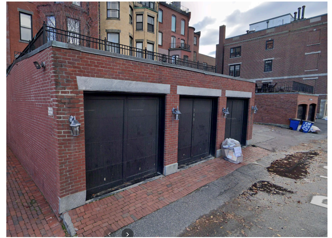
348 / 352 BEACON STREET REAR GARAGE WITH ROOF DECK
