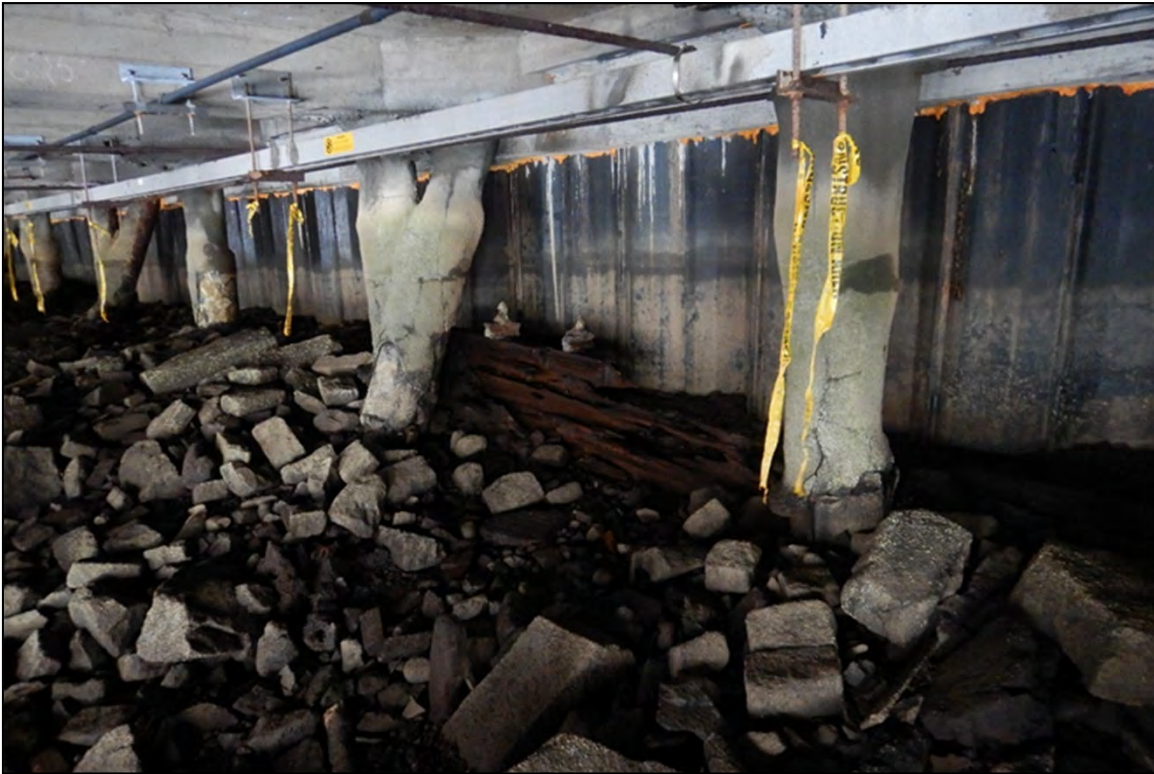
Photo 11 – Overview of the bulkhead and riprap slope beneath Wharf 3.
