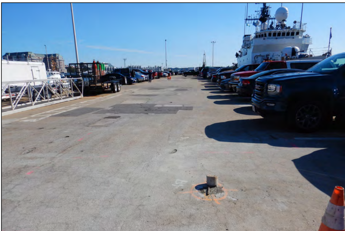
Photo 2 – Overview of Pier 2 looking east.
