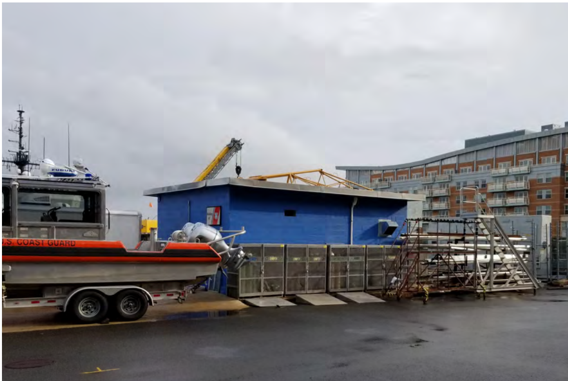
Photo 27 – View of the exterior of Building 7.
