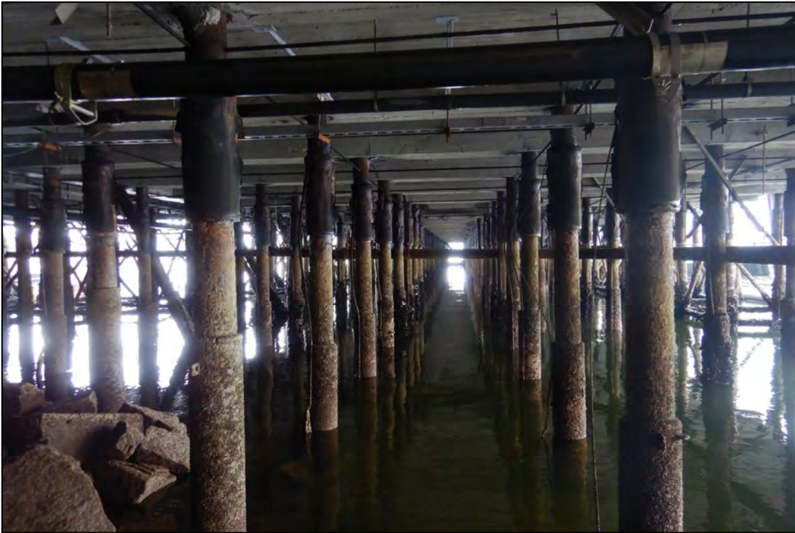
Photo 21 – Typical view of the support piles beneath Wharf 3/Pier 2 looking east.
