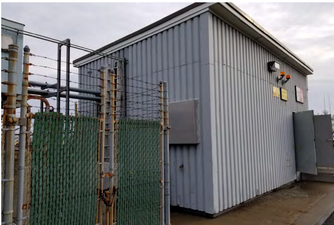
Photo 28 – View of the exterior of Building 11.
