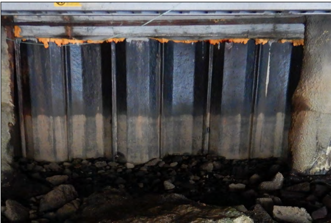
Photo 12 – Typical condition of the bulkhead beneath Wharf 3.
