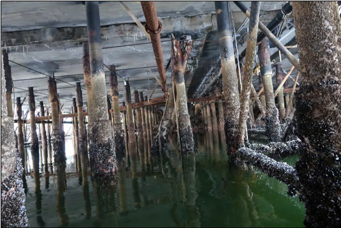
Photo 23 – View of the Pier 2 support piles and utilities looking west.
