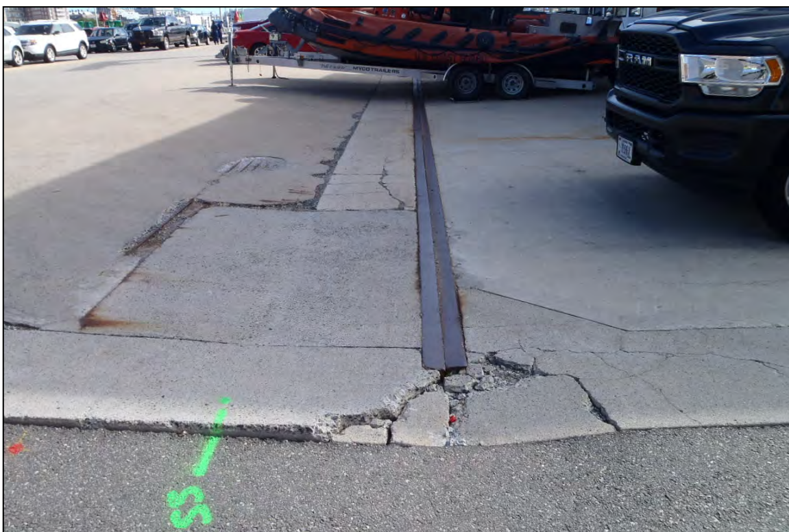
Photo 8 – View of the joint along south side of Wharf 3 looking east.
