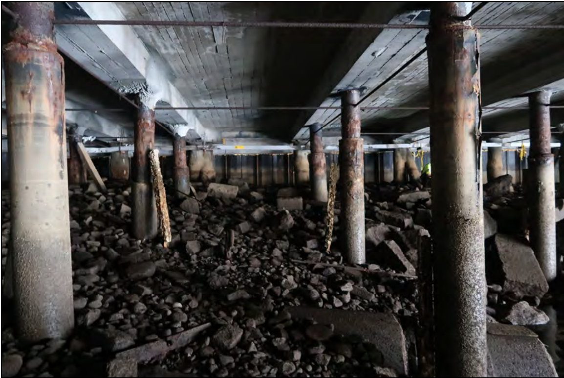
Photo 17 – View riprap slope at the western end of Wharf 3 looking north.
