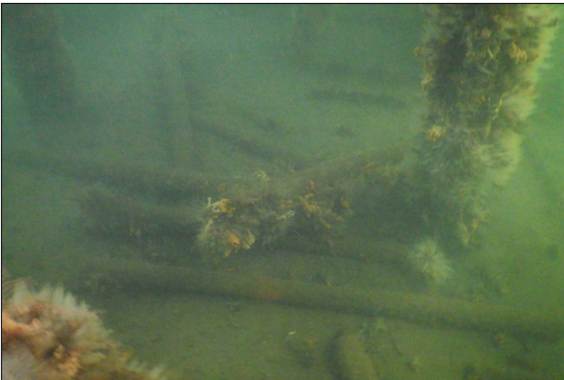
Photo 26 – Typical underwater conditions showing typical pile condition and debris.
