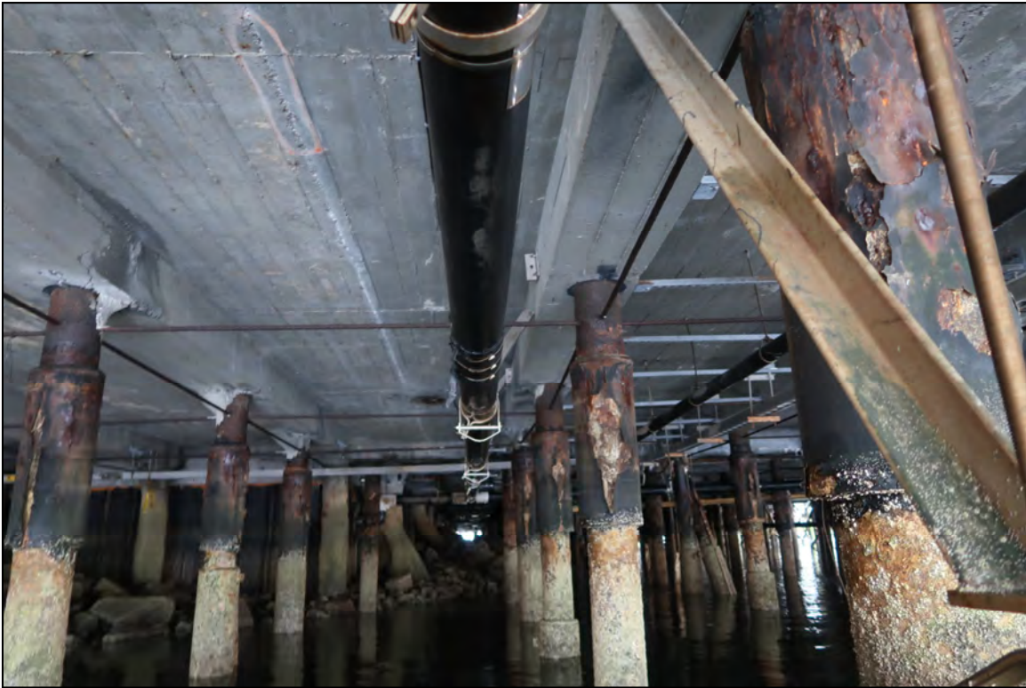
Photo 19 – View of the underside of Wharf 3.
