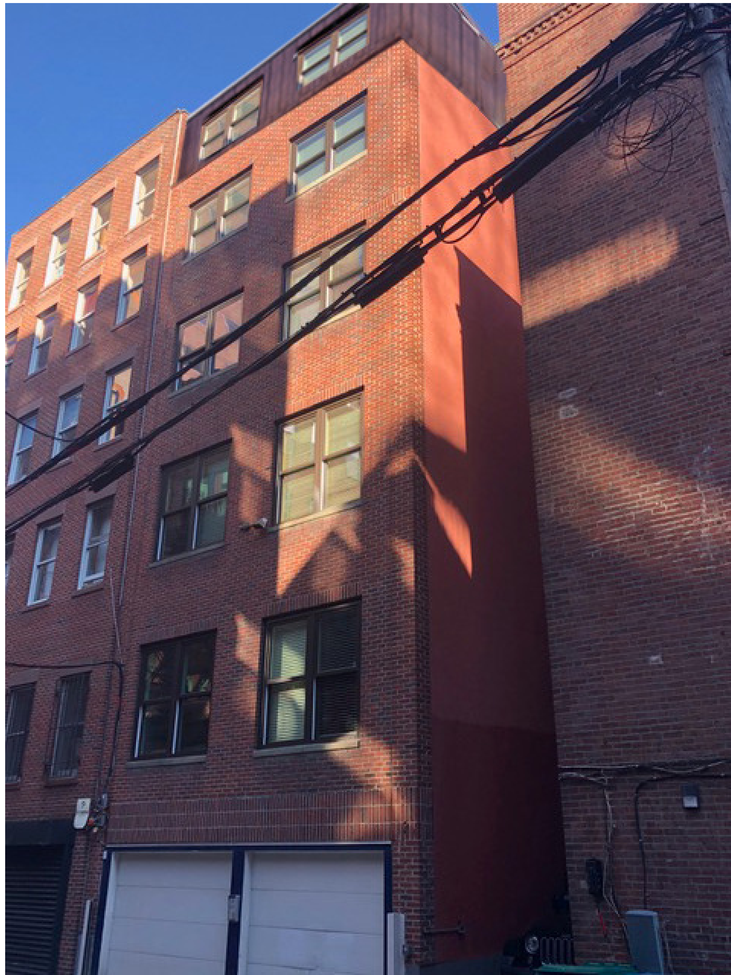
2 EXISTING REAR FACADE 1 1/2" = 1'-0"
