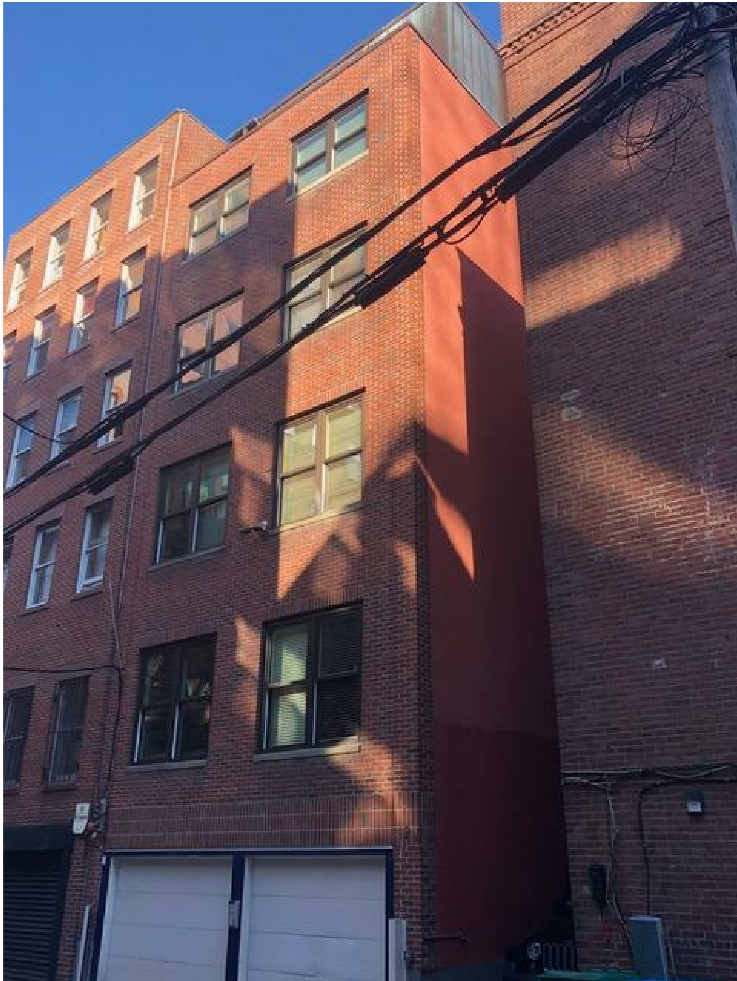
1 EXISTING REAR FACADE 1 1/2" = 1'-0"
