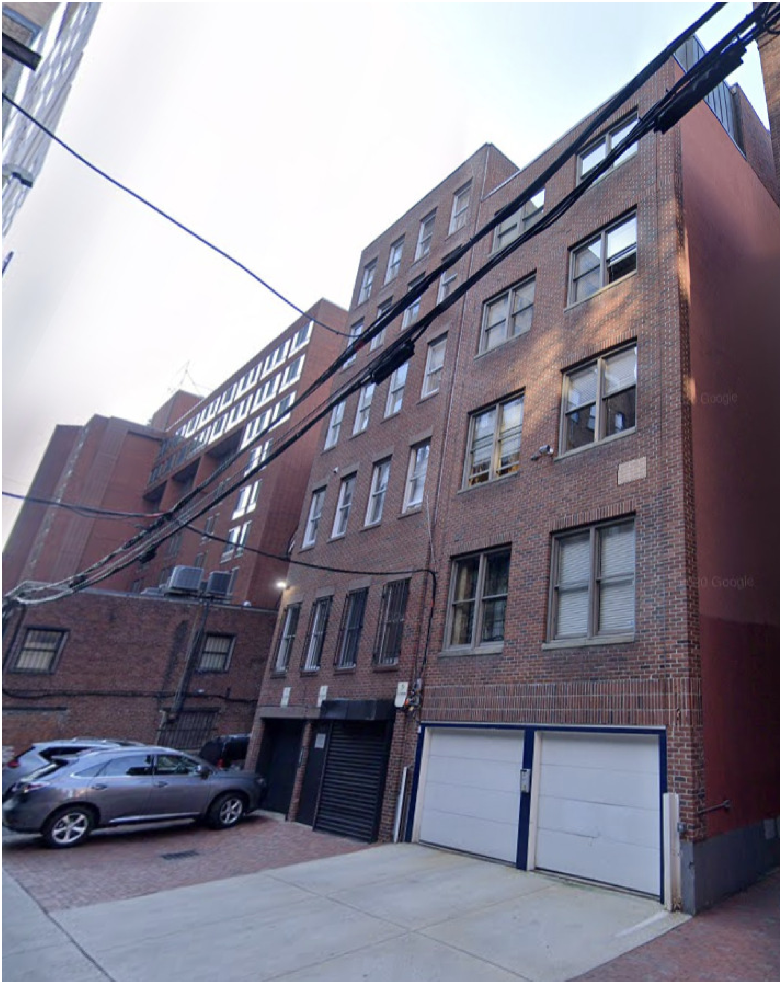
2 EXISTING REAR FACADE 1 1/2" = 1'-0"
