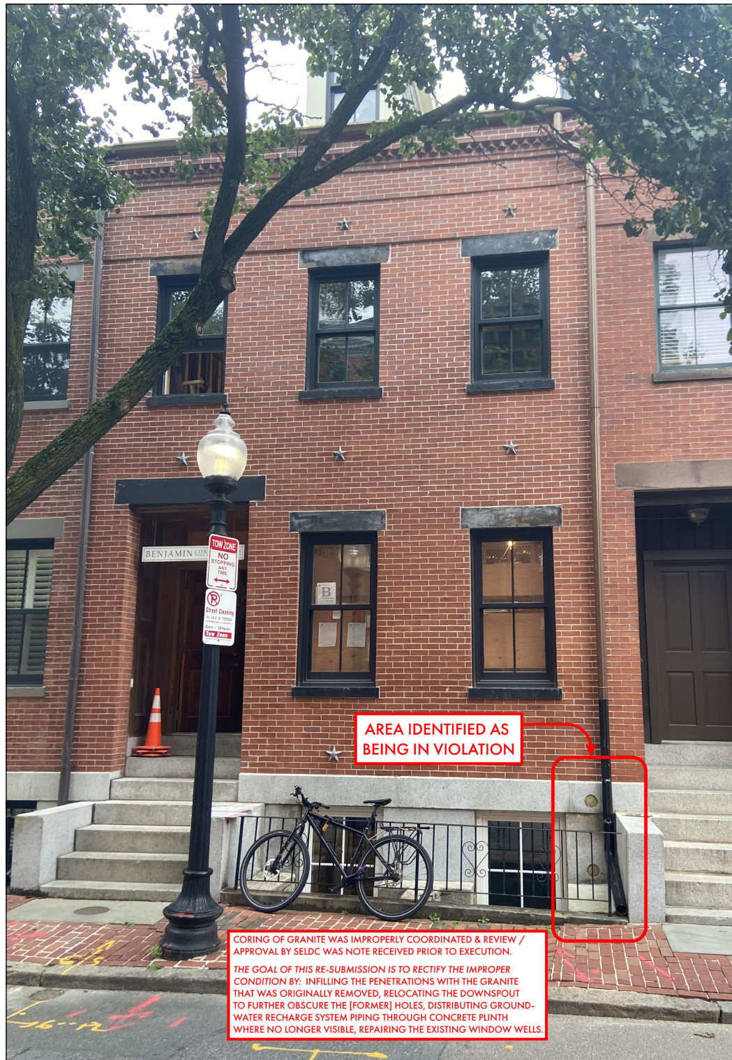
1 3 BOND VIEWED FROM OPPOSITE SIDE OF STREET
