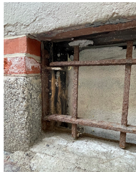
EXISTING PREVIOUSLY INFILLED BASEMENT WINDOWS
