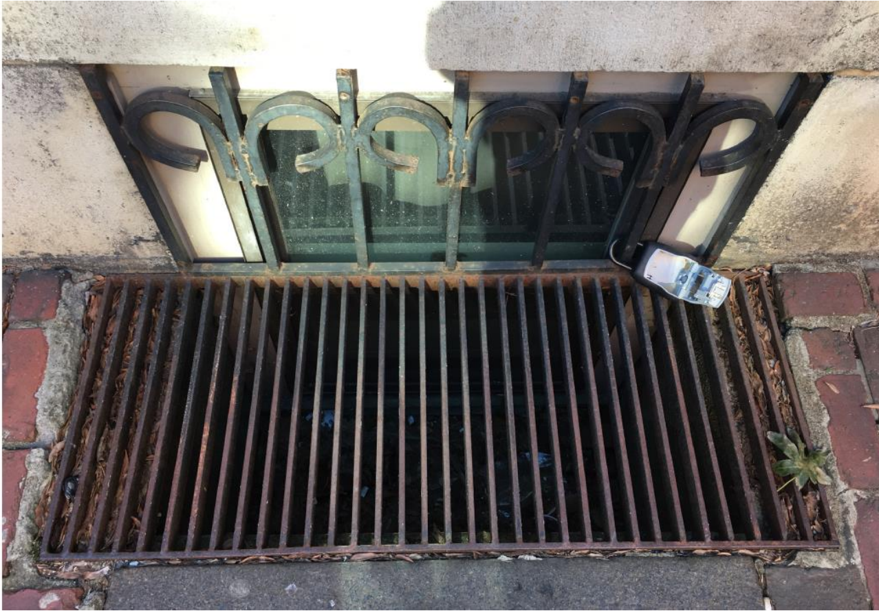
Subject Window – sidewalk bar grating to remain
