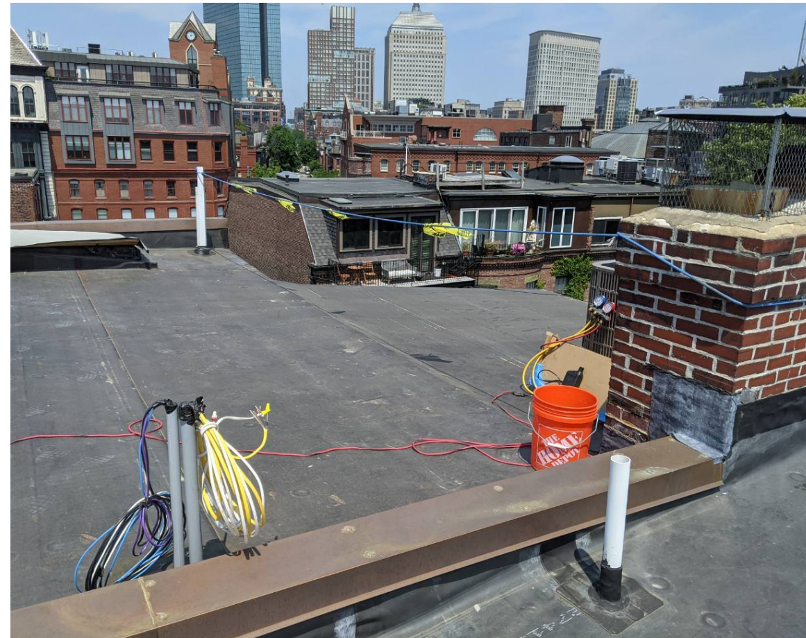
ROOF DECK MOCK-UP
