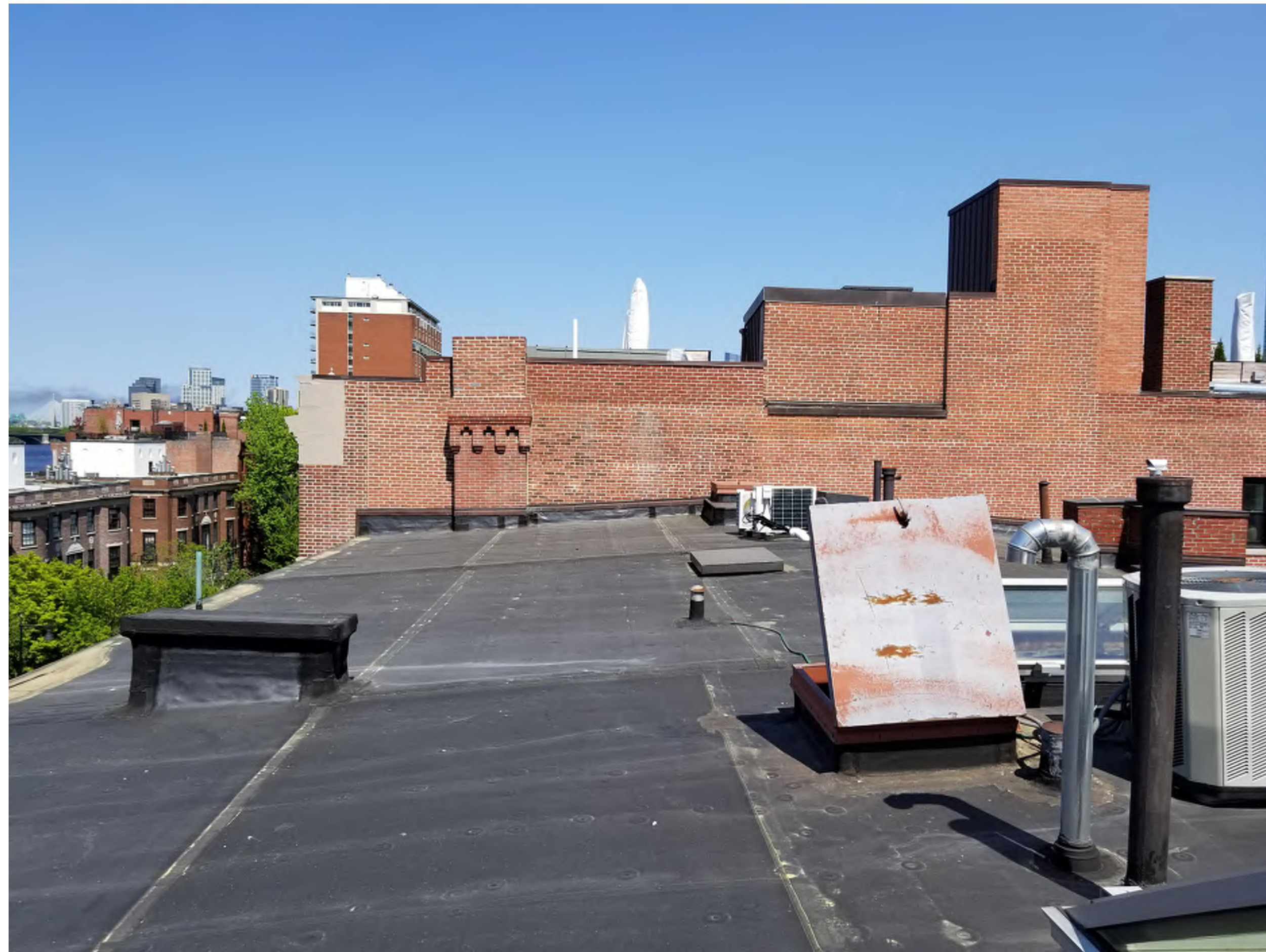
LOOKING NORTH-EAST TOWARDS 405 BEACON
