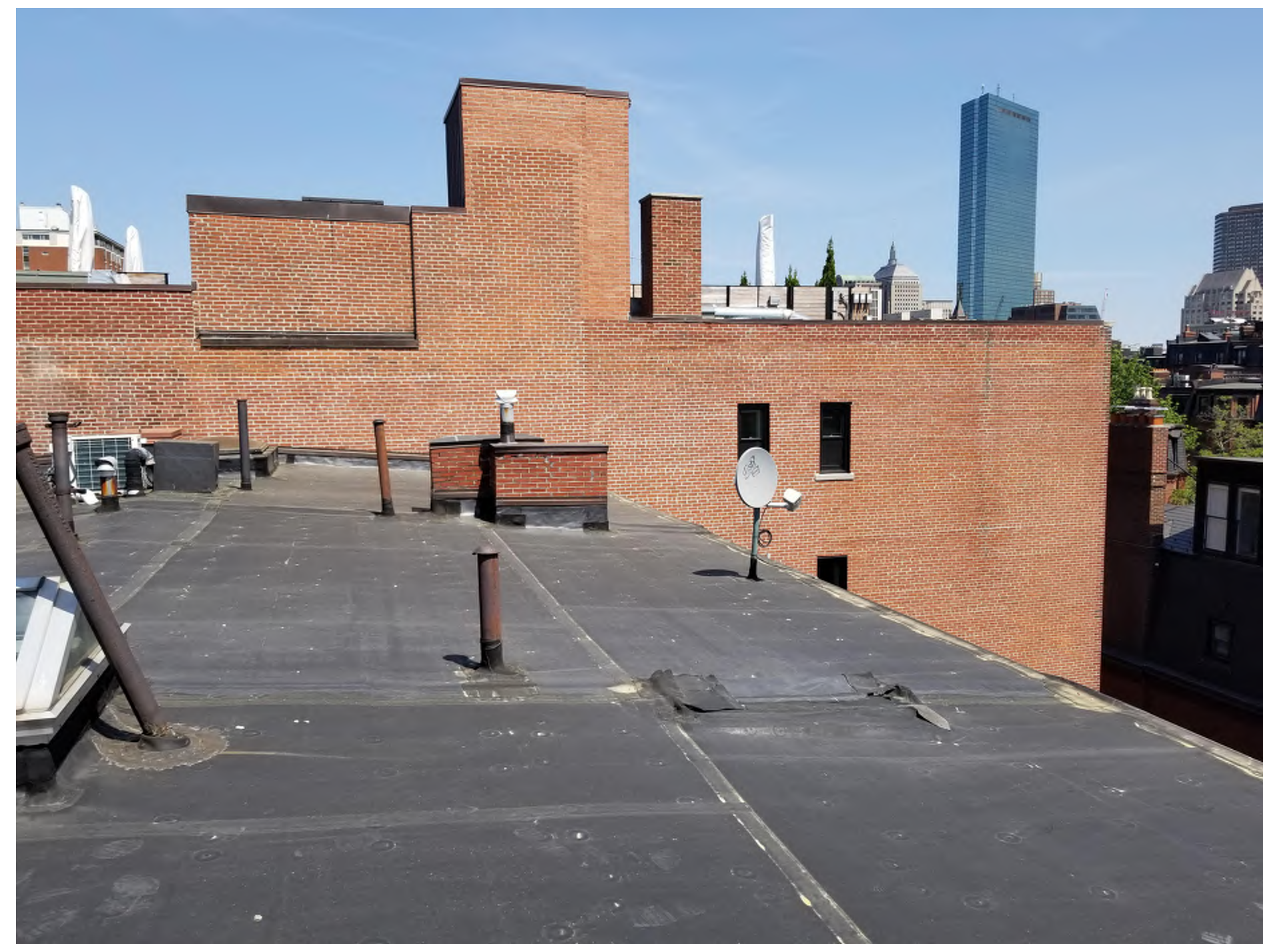
LOOKING NORTH-EAST TOWARDS 405 BEACON
