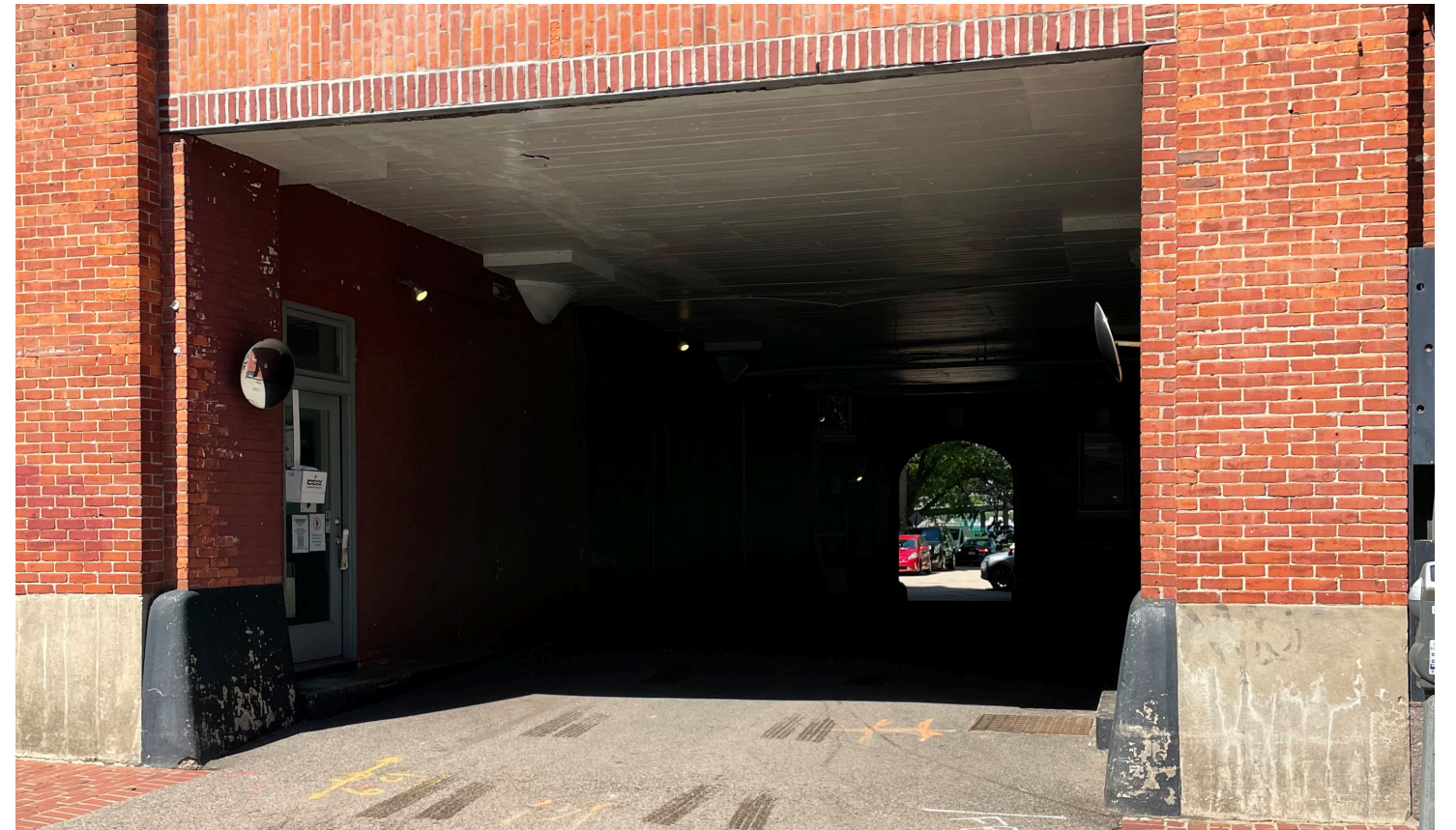
EXISTING VIEW LOOKING WEST
