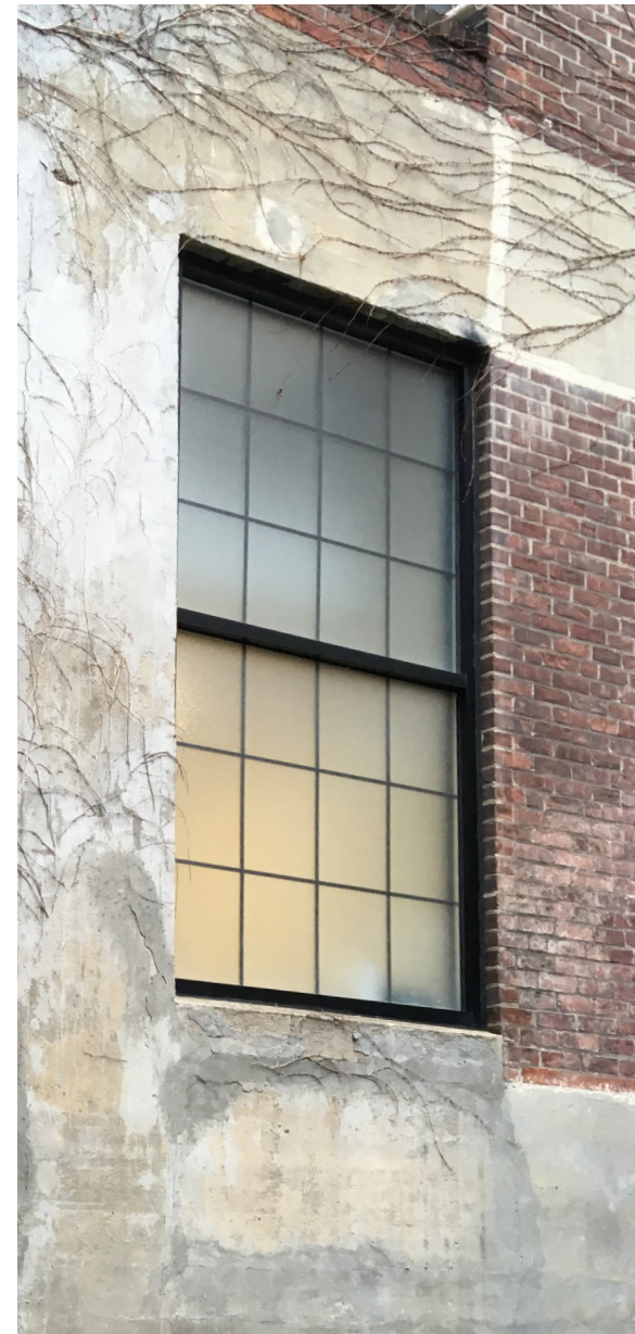
Existing windows with translucent film on south facade
