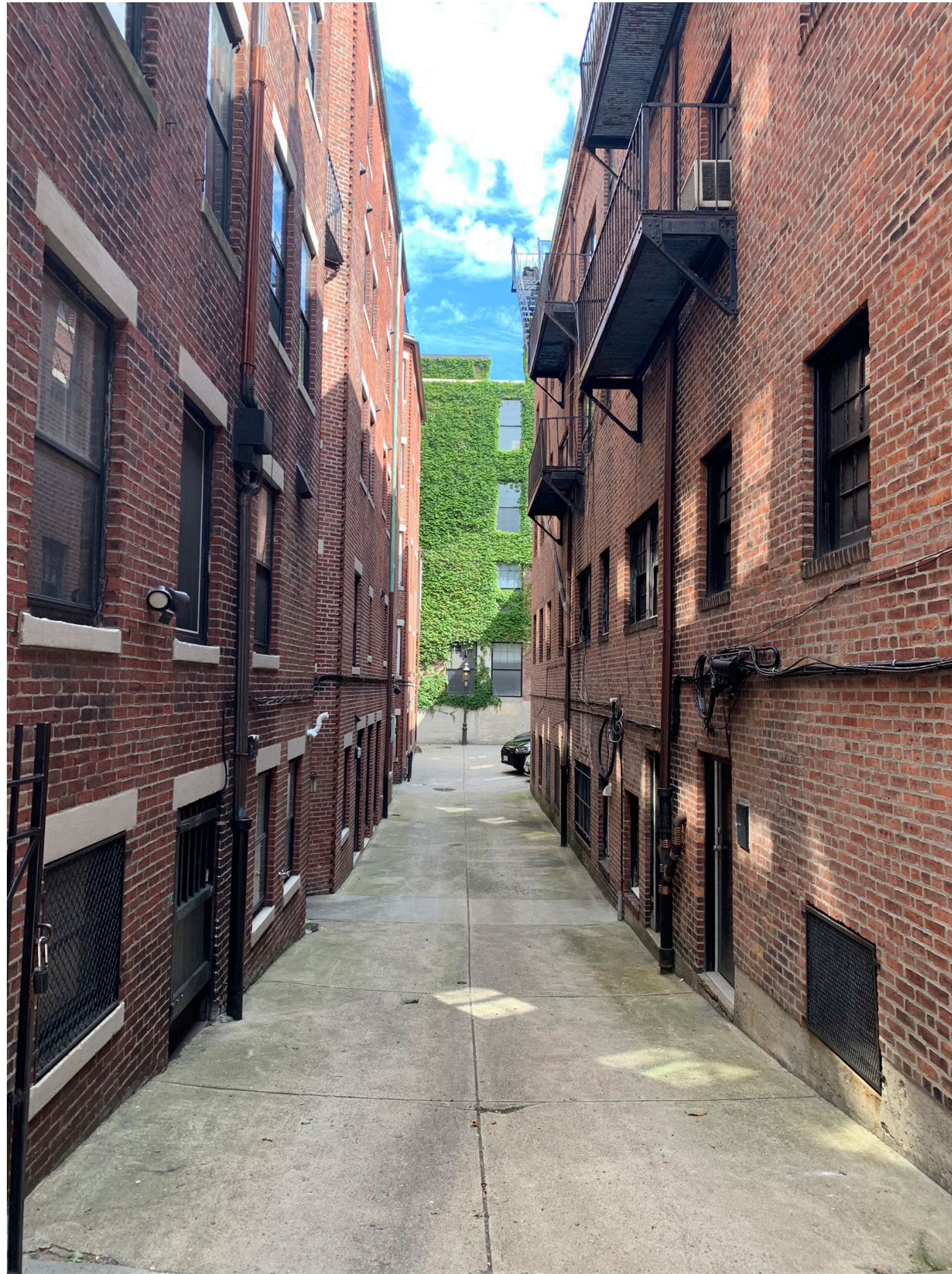
View from Revere Street looking north
