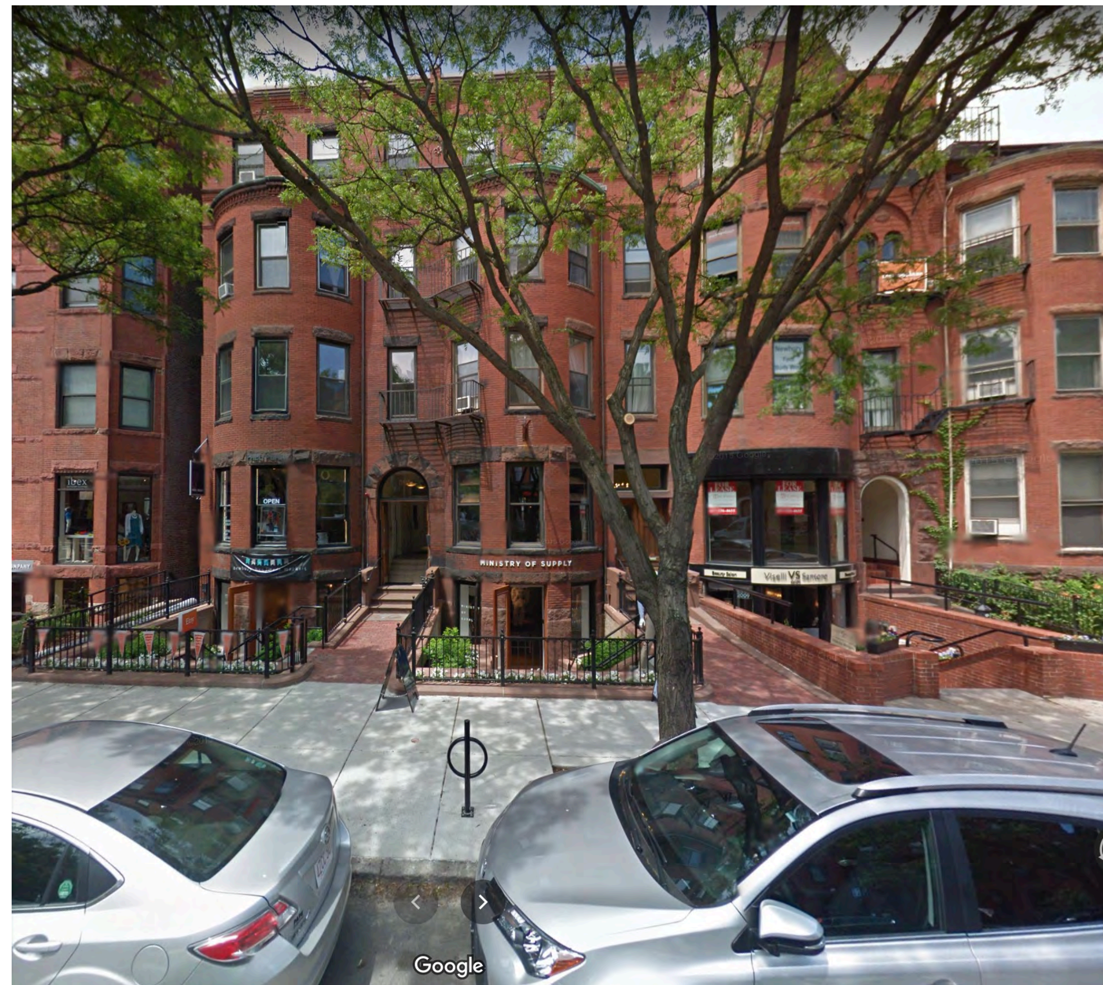
EXISTING NEWBURY STREET FACADE
