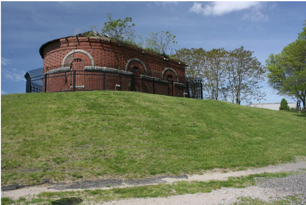
Figure 14. West Shaft Entrance
