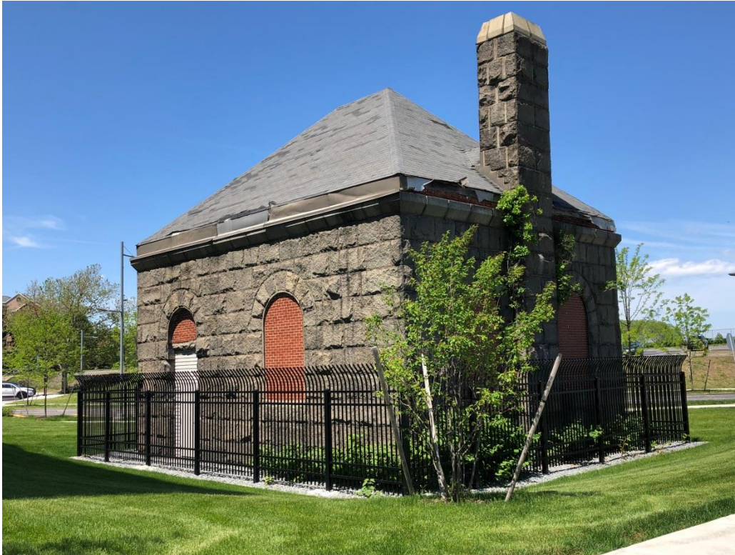
Figure 9. Gate House-Filth Hoist
