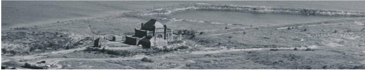
Historic Image 12. Aerial View, 1946 (UMB Histories of the Calf Pasture Pumping Station)
