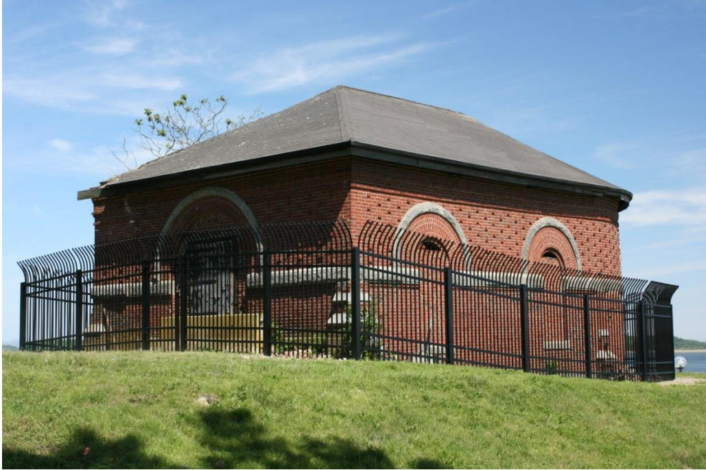
Figure 13. West Shaft Entrance
