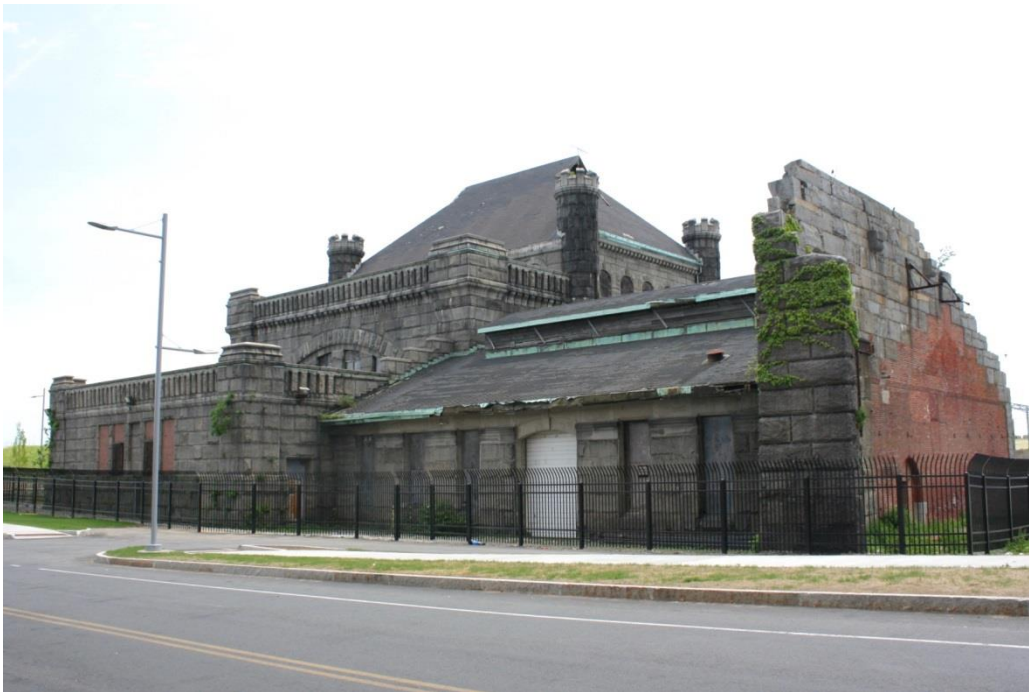
Figure 4. Pumping Station-Engine House and Boiler House
