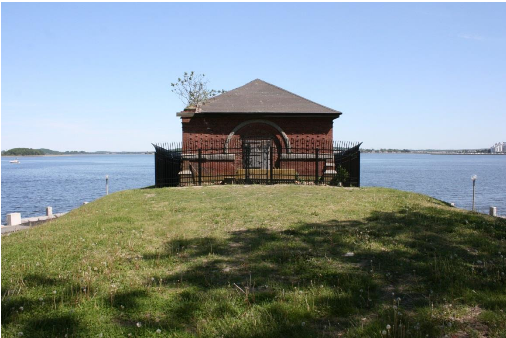
Figure 12. West Shaft Entrance
