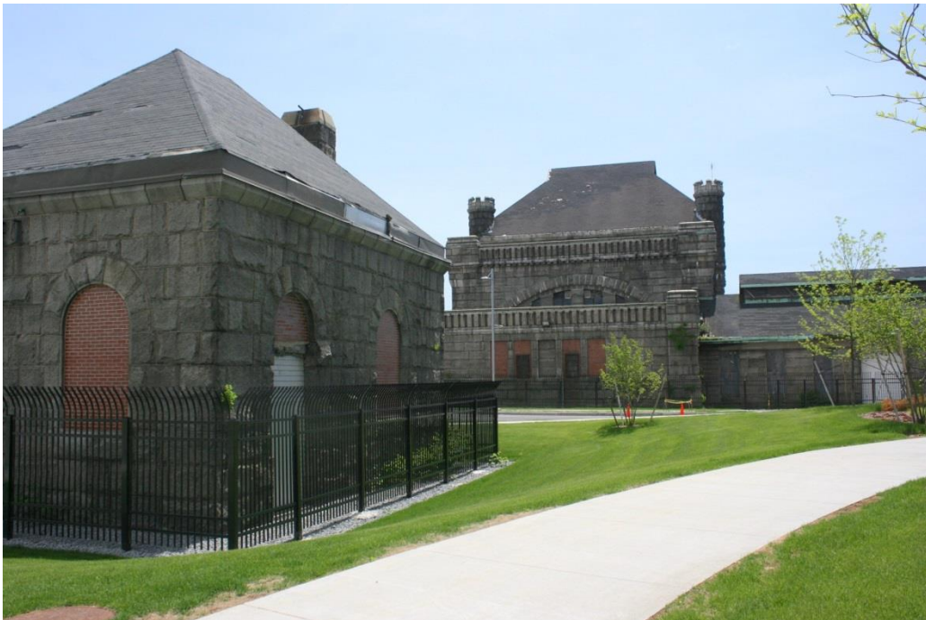
Figure 8. Gate House-Filth Hoist and Pumping Station
