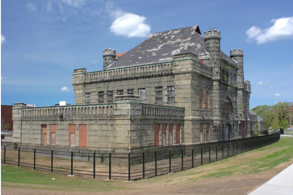
Figure 2. Pumping Station Engine House
