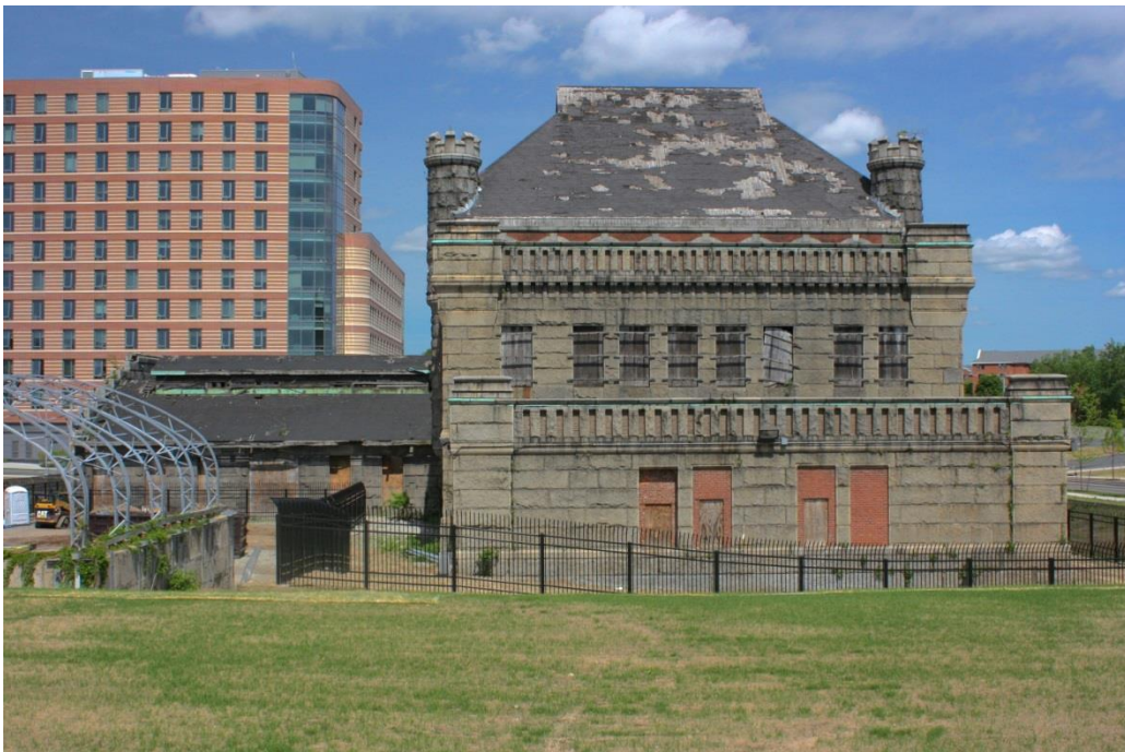
Figure 6. Pumping Station-Boiler House and Engine House
