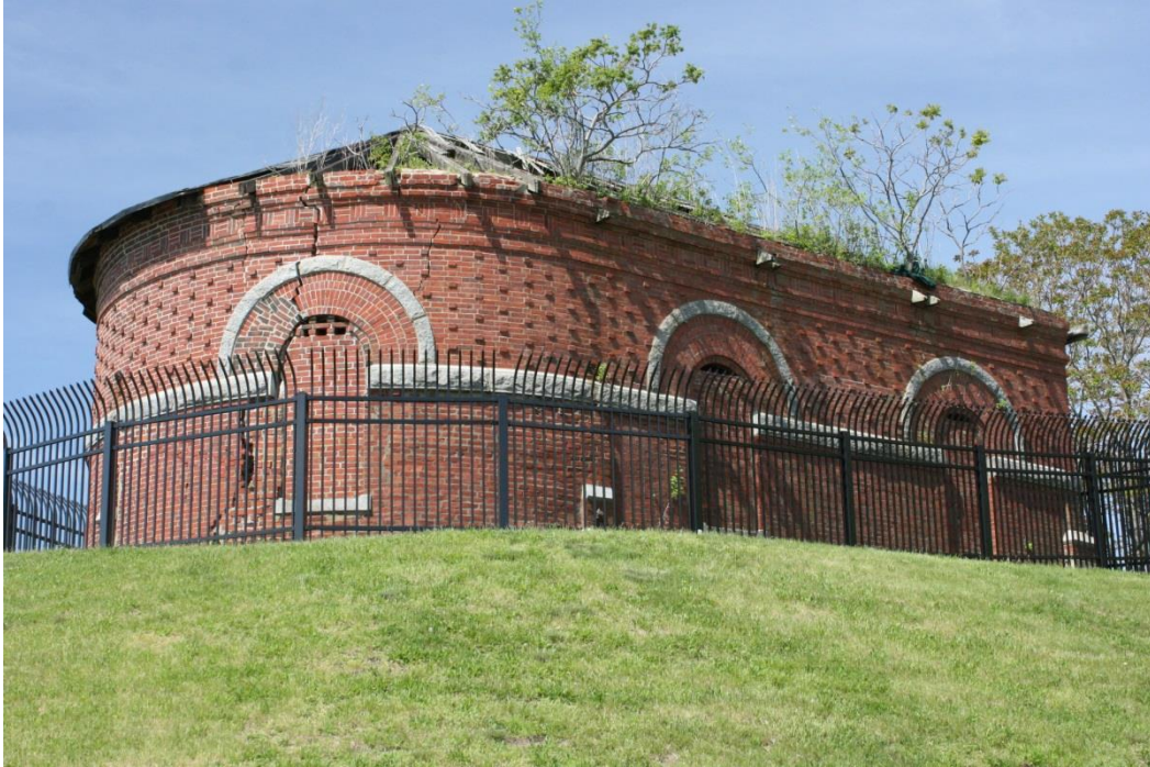
Figure 15. West Shaft Entrance
