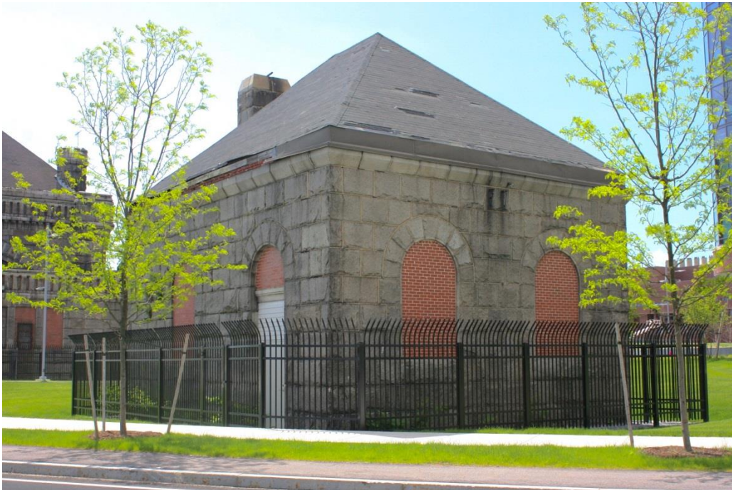
Figure 10. Gate House-Filth Hoist
