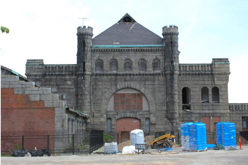
Figure 5. Pumping Station-Boiler House and Engine Room
