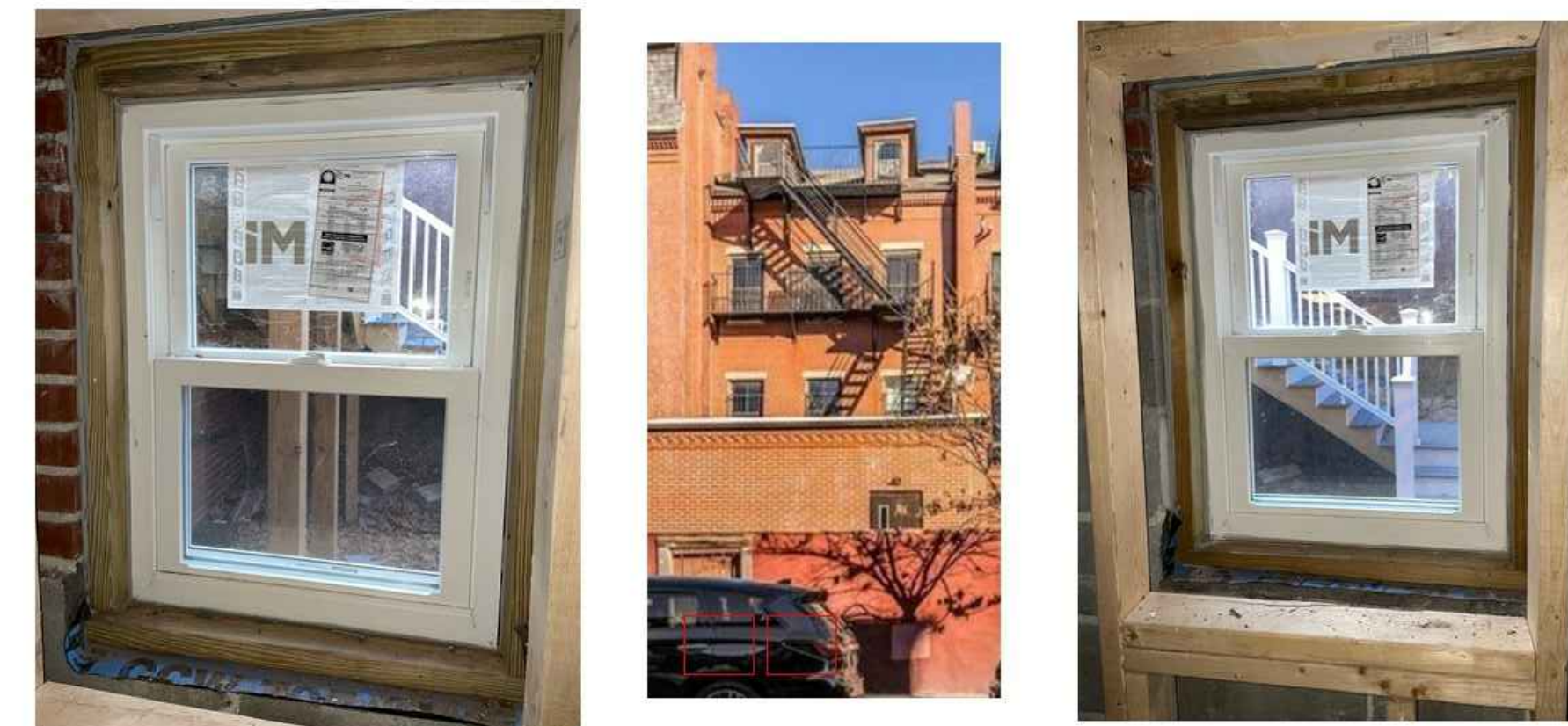
Interior Photos – Garden Level Backyard
