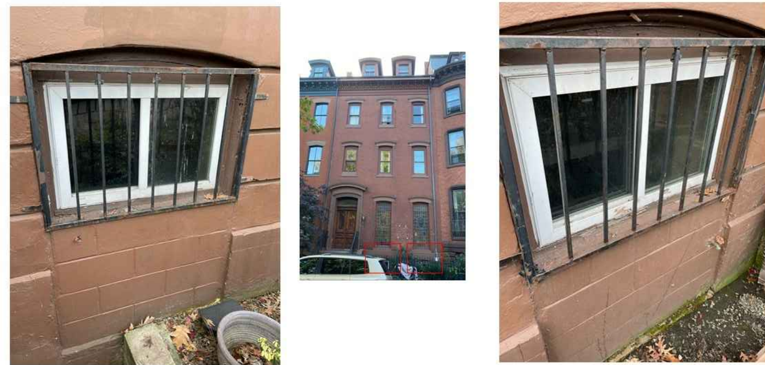
Exterior Photos – Garden Level Front
