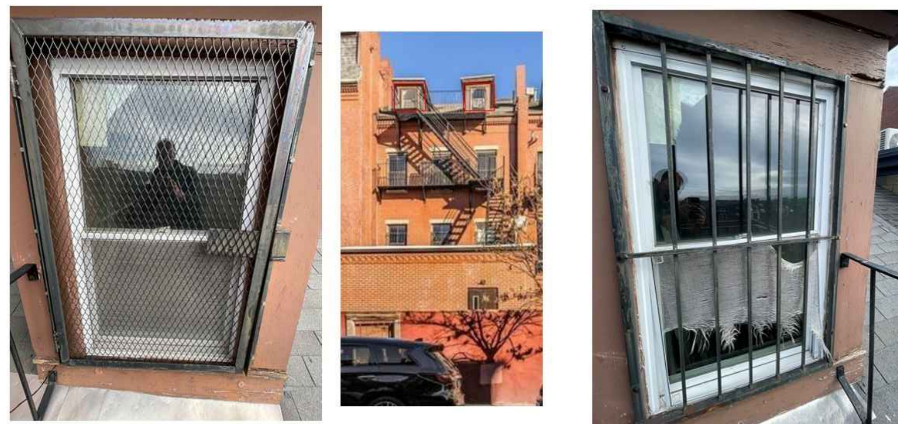
Exterior Photos – 4th Floor Backyard
