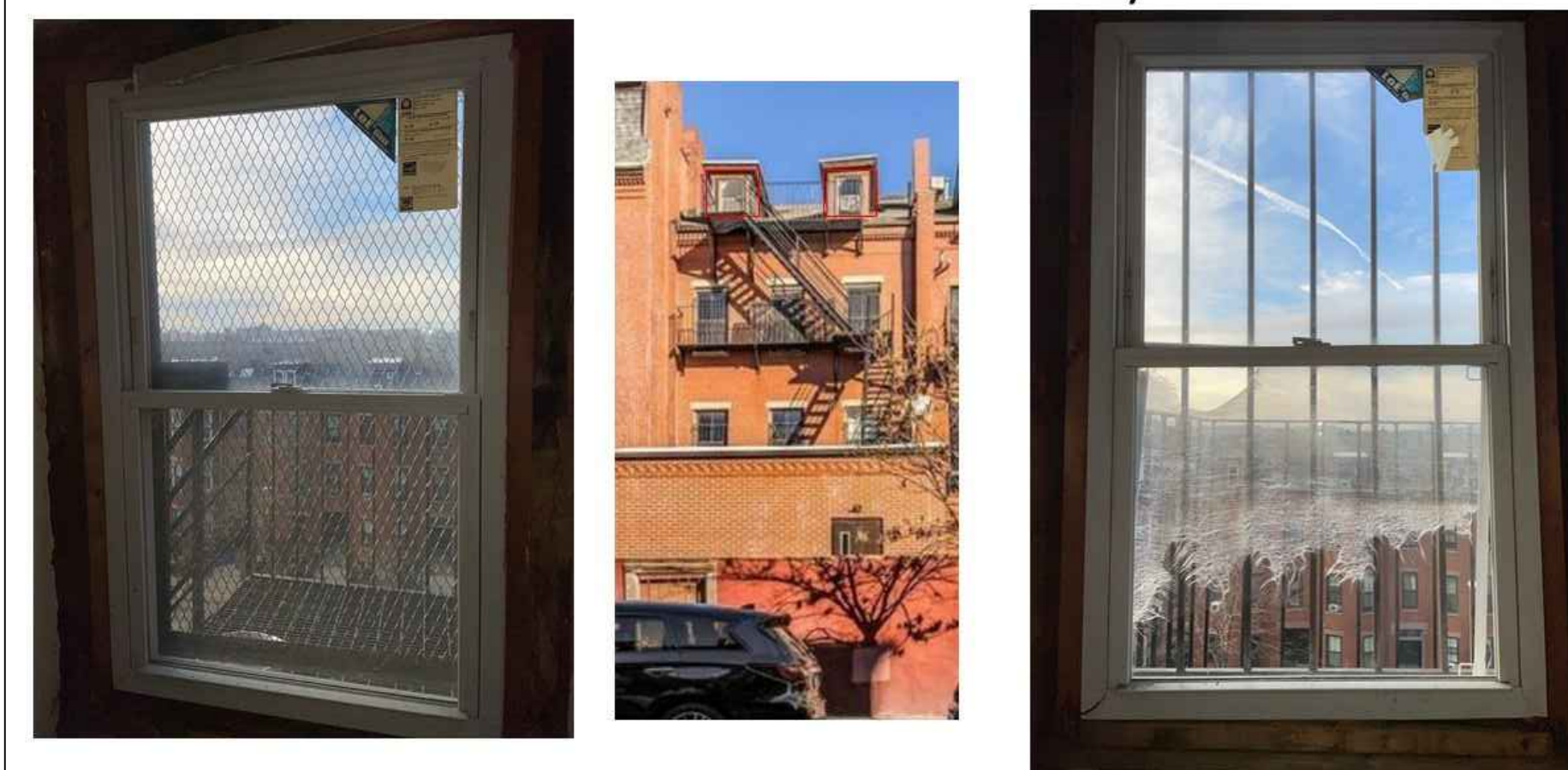
Interior Photos – 4th Floor Backyard
