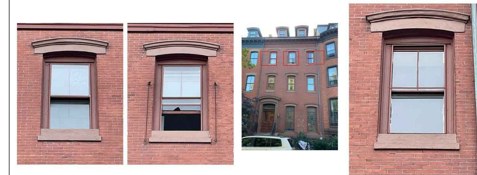
Exterior Photos – 3rd Floor Front
