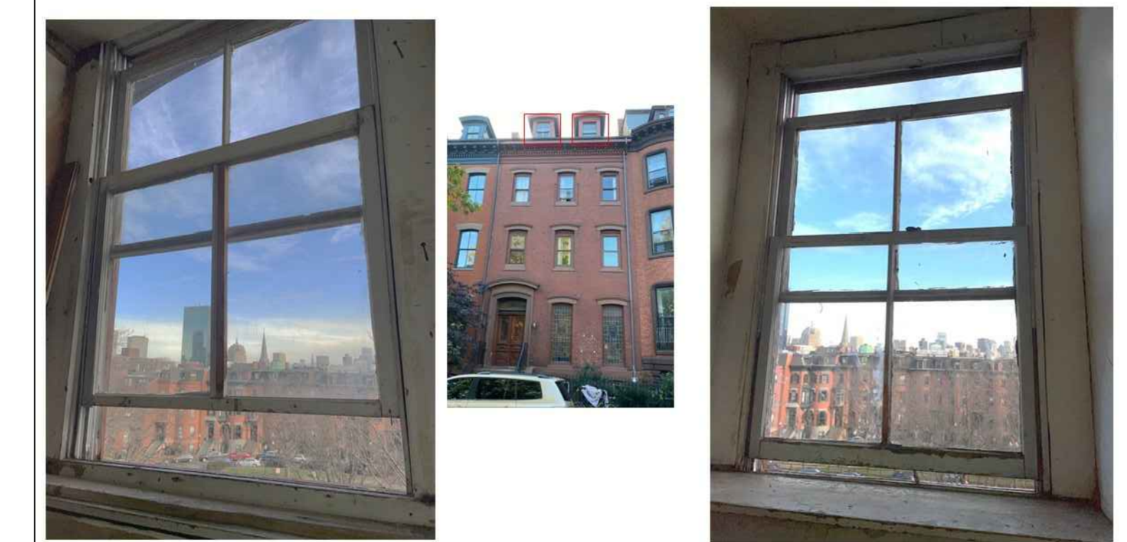
Interior Photos – 4th Floor Front
