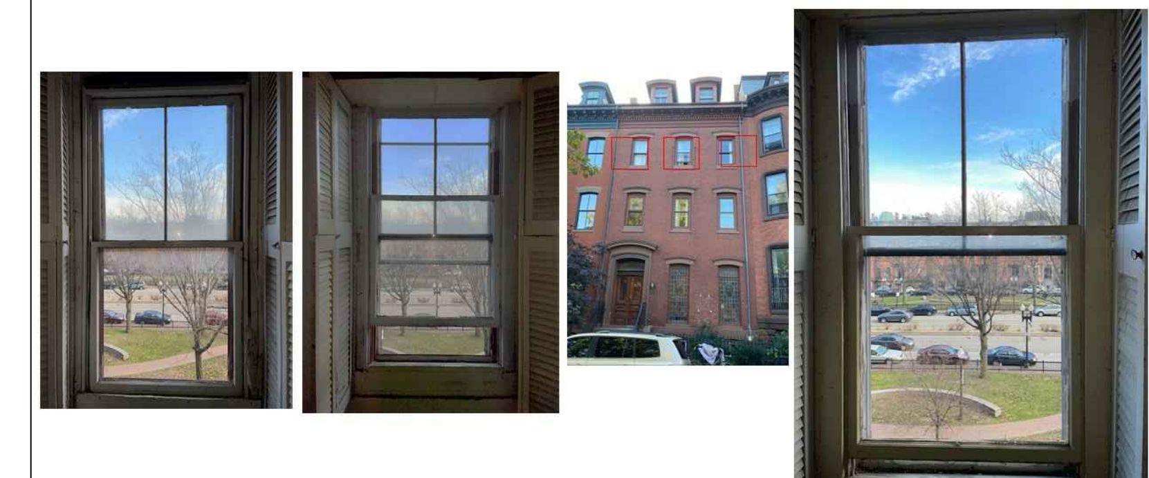
Interior Photos – 3rd Floor Front
