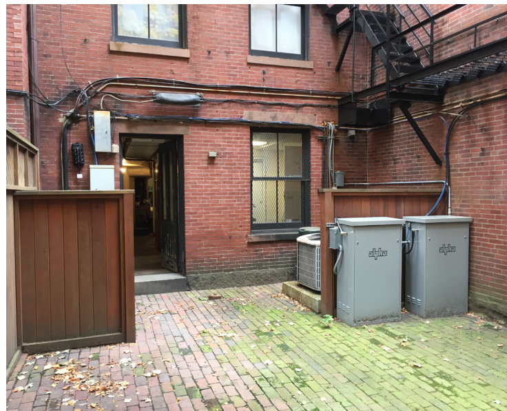
EXISTING COURTYARD + COMCAST BOXES
