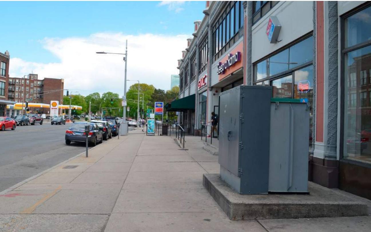
BOYLSTON STREET EXISTING CONDITION
