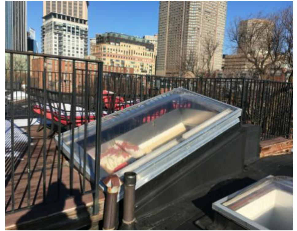
EXISTING ROOF HATCH
