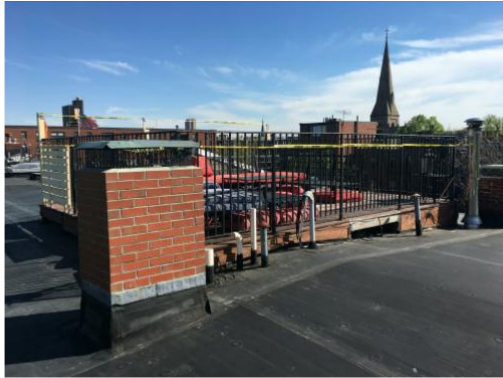
VIEW NORTH FROM ADJACENT ROOF
