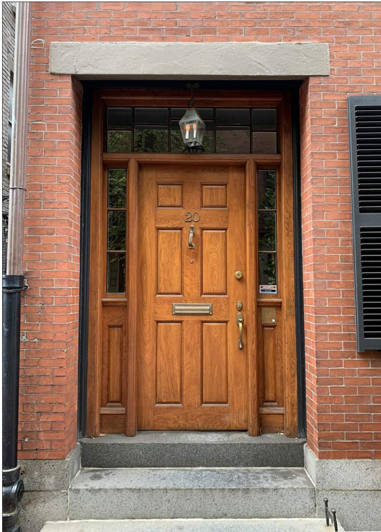
1 EXISTING VIEW 1 - FRONT ENTRY (VISIBLE FROM WEST CEDAR STREET)
