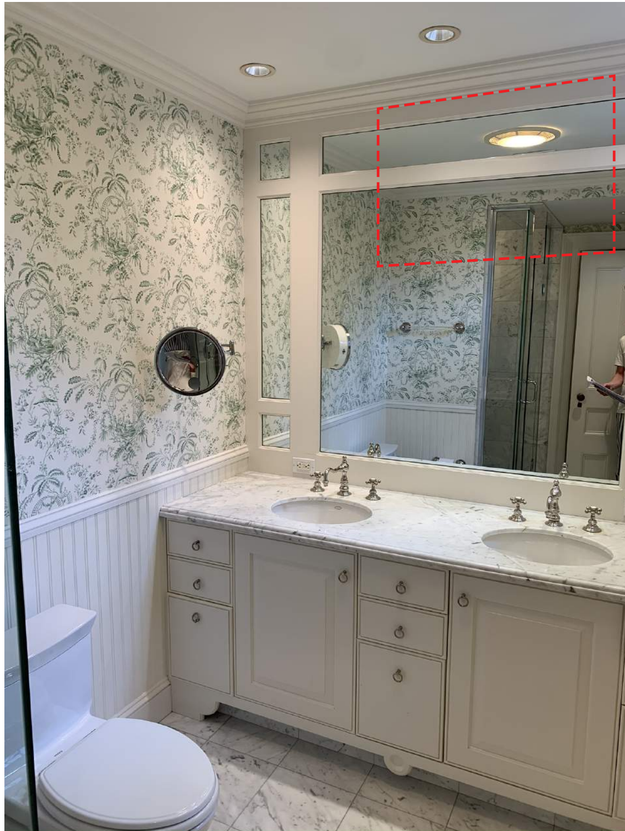
MIRROR TO BE REMOVED TO REVEAL EXISTING WINDOW (UNIT 16 DASHED IN RED) BEYOND. WINDOW TO REMAIN & BE REPAIRED AS NEEDED.
