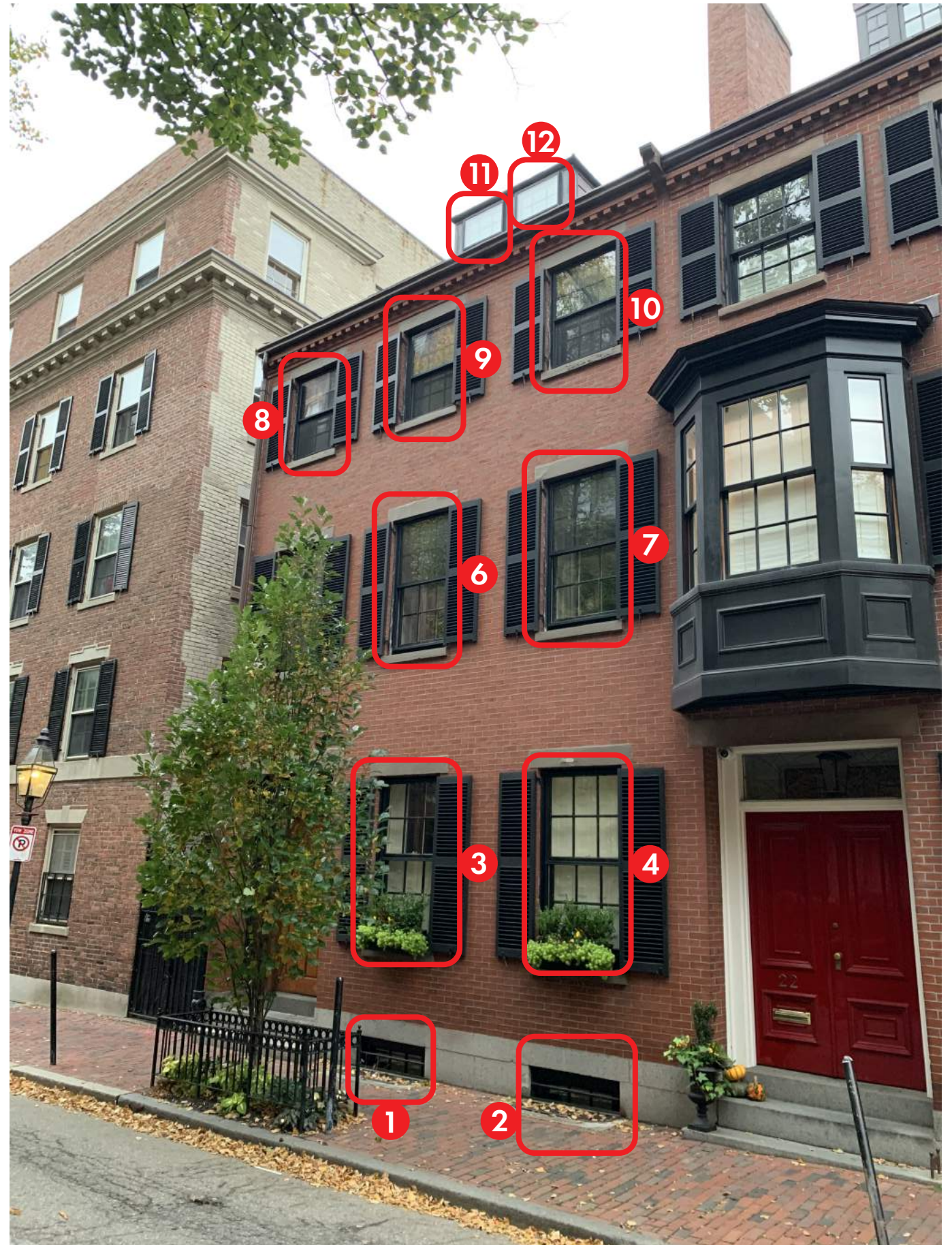
FRONT FACADE, EAST-FACING WINDOWS
