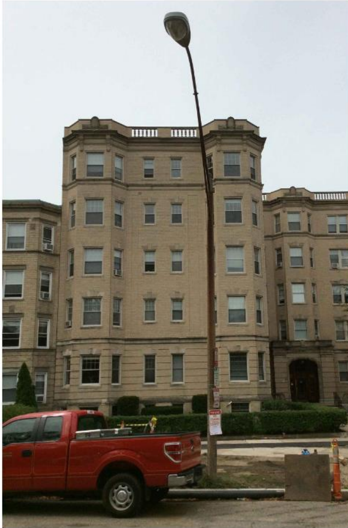
EXISTING PHOTOGRAPHIC VIEW 42.343889°, -71.094967°
