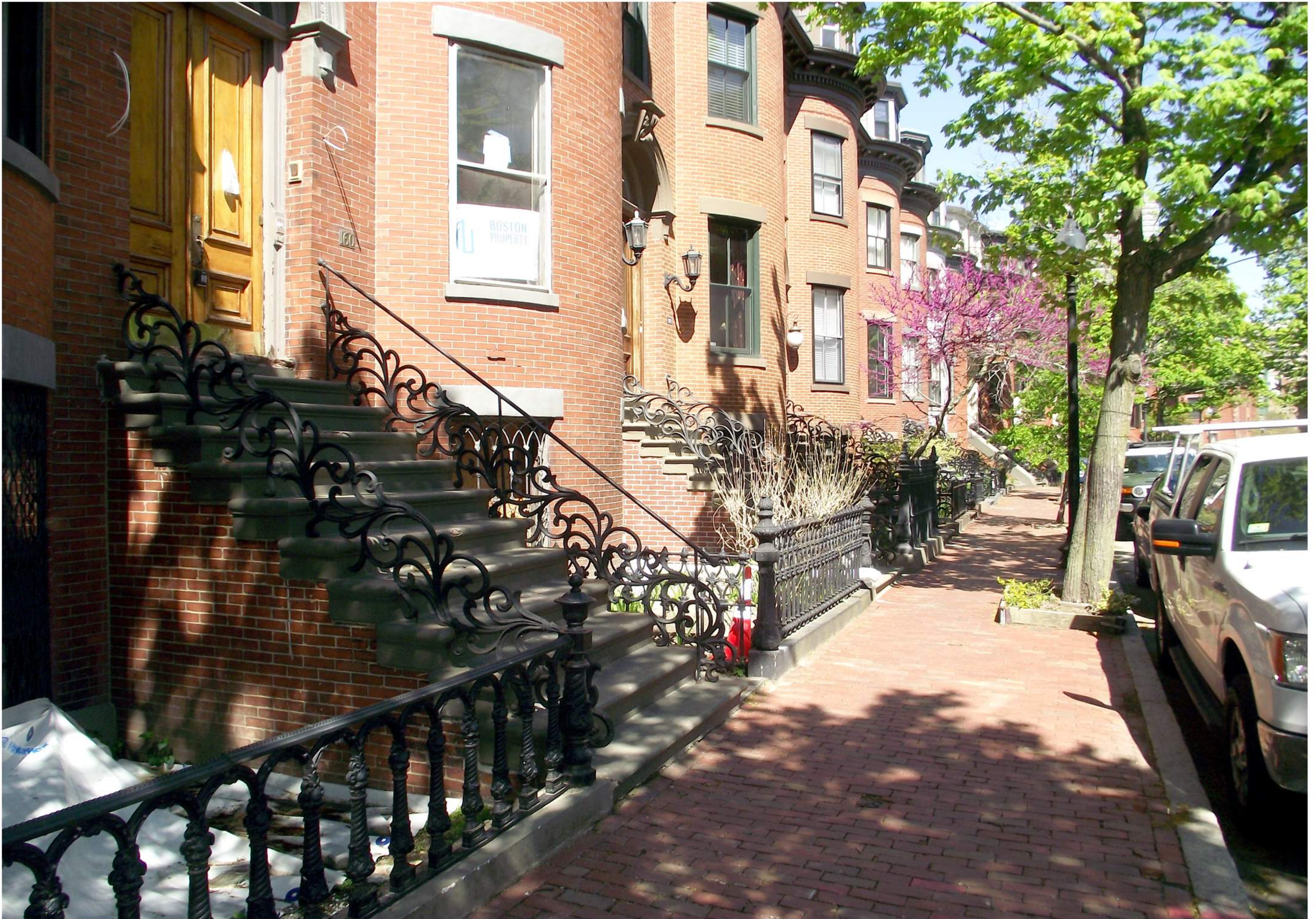
158 West Canton Street: Decorative Metal Railings Railing precedents at neighboring buildings (160 - 170 West Canton)
