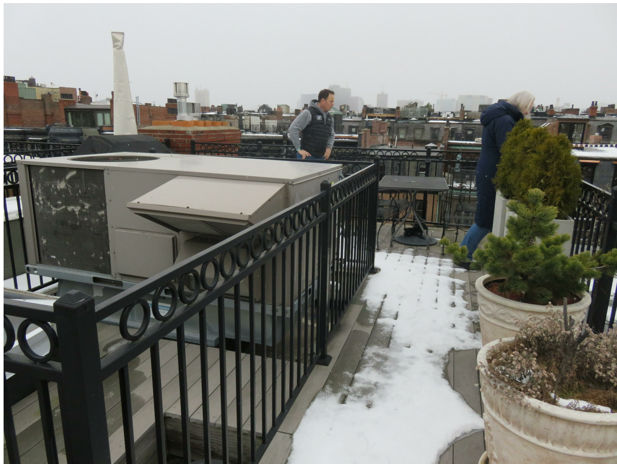
EXISTING ROOF DECK - MECHANICAL
