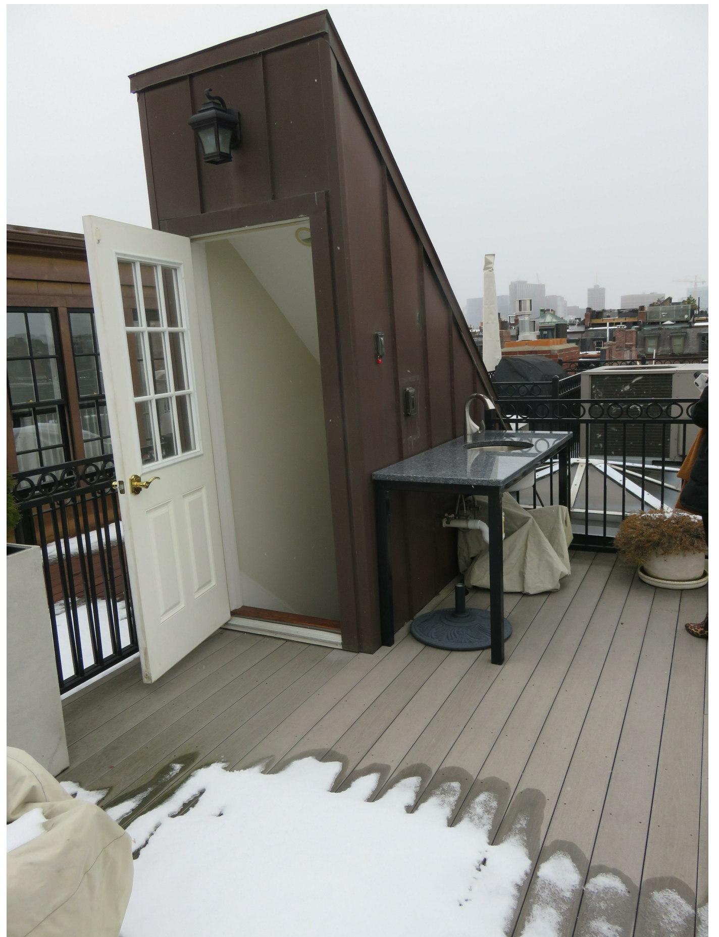
EXISTING ROOF DECK - HEADHOUSE
