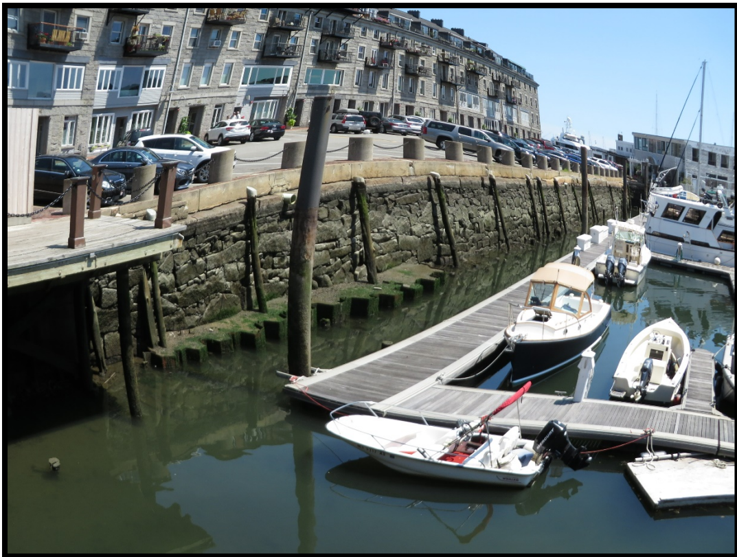
Photograph 2. South Boardwalk Site Stone Bulkhead
