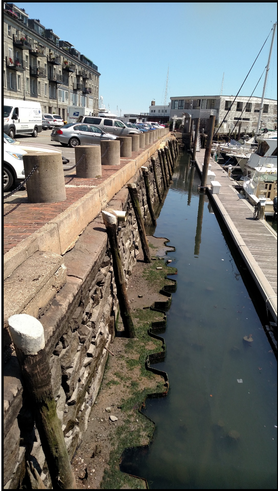
Photograph 3. Existing South Boardwalk Site Looking East
