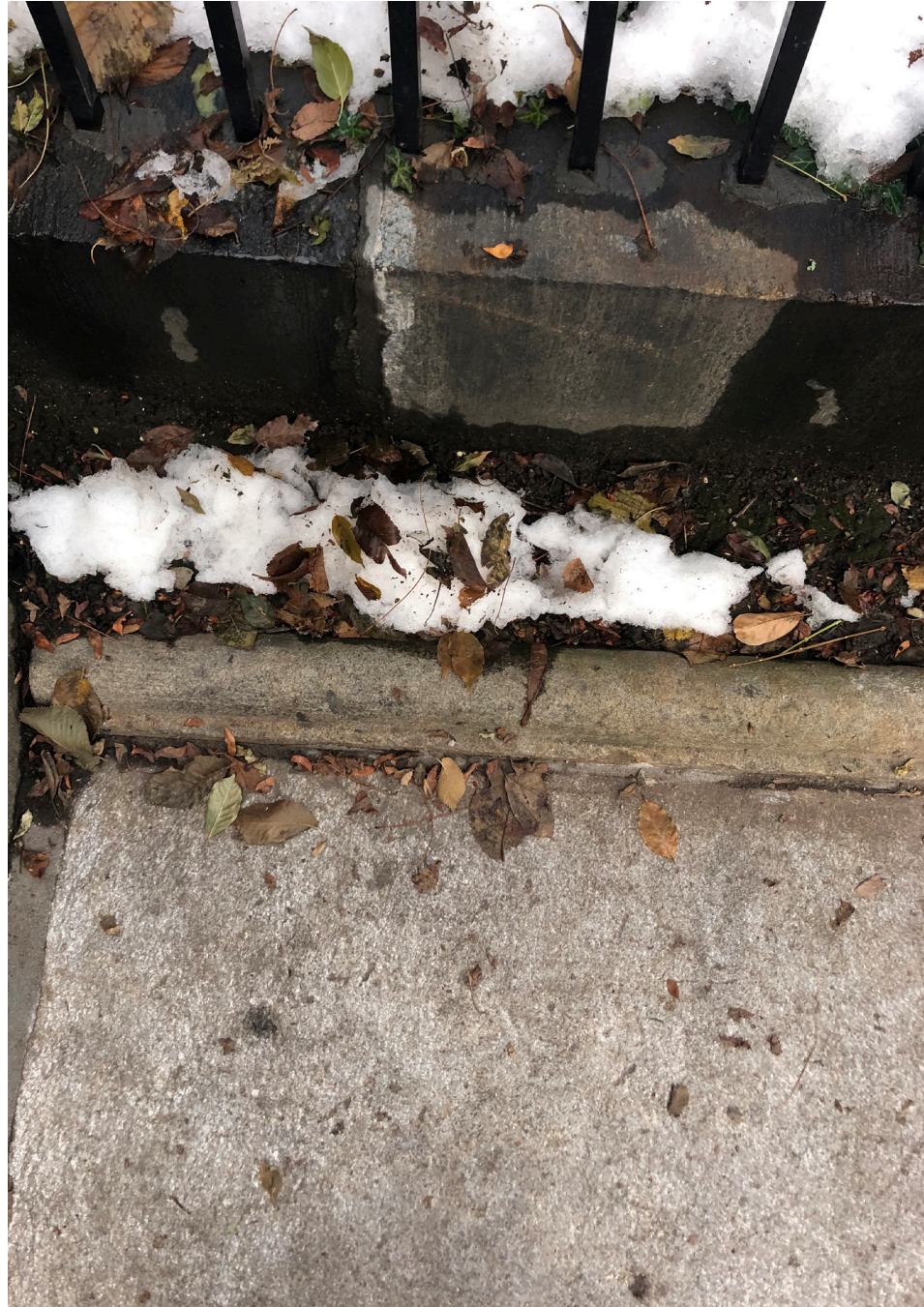
Close up of existing granite paving
