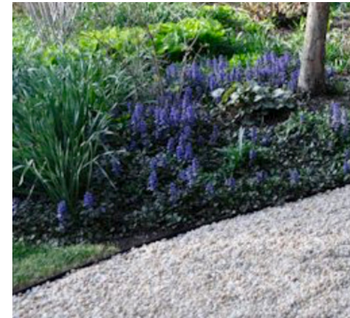
A metal retaining edge keeps peastone from migrating into the plant beds
