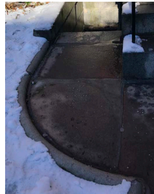
Granite paving with 1/2 round edging to be mirrored at stairs for bench landing
