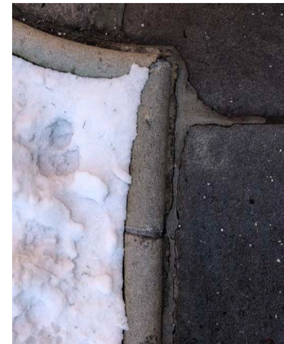
Close up of 1/2 round granite edging to be replicated
