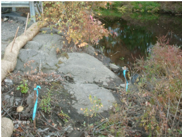
North Corner of property at paved outfall from Storage/ parking area.
