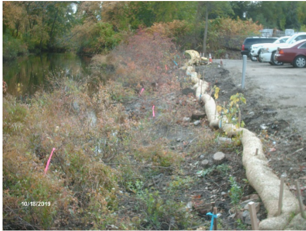
Looking south along rear of property.
