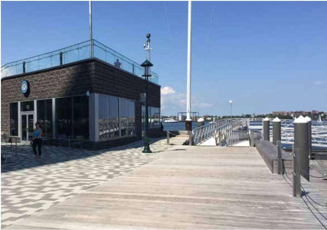
Harborwalk and gangway in the northwestern portion of the Project Site
