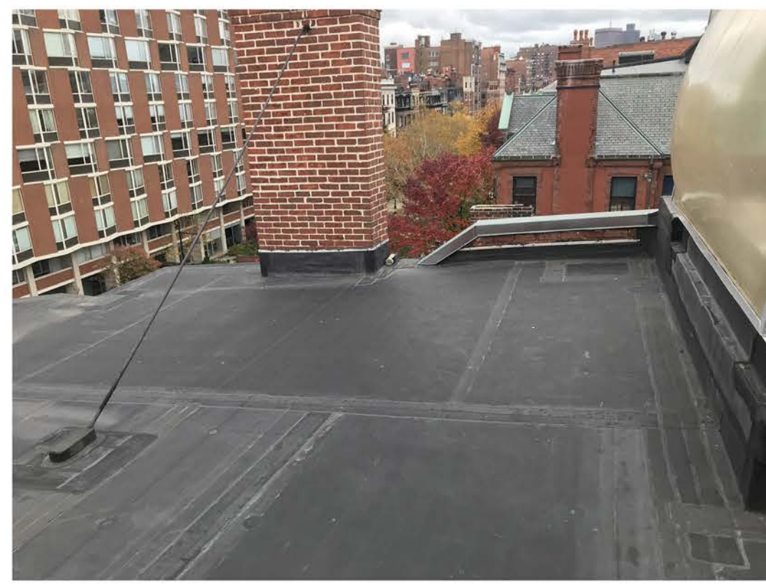
EXISTING FRONT ROOF
