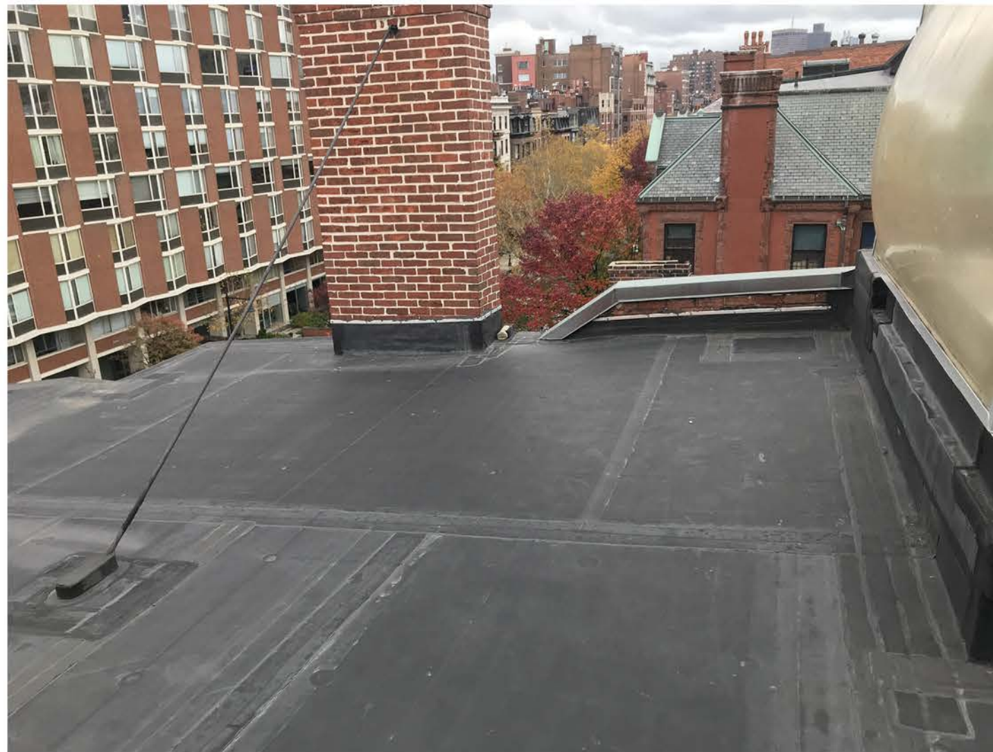
EXISTING FRONT ROOF
