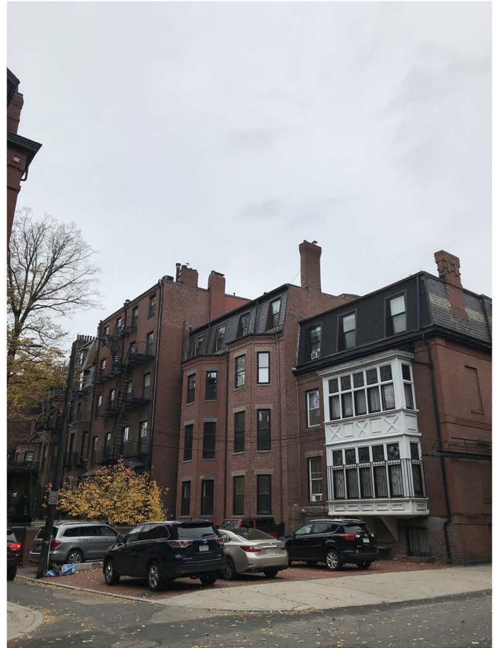
VIEW FROM FAIRFIELD STREET - REAR
