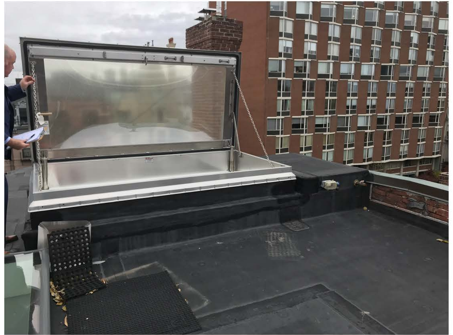
EXISTING ROOF HATCH
