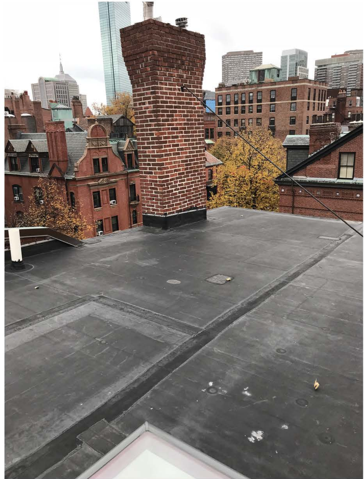
EXISTING REAR ROOF
