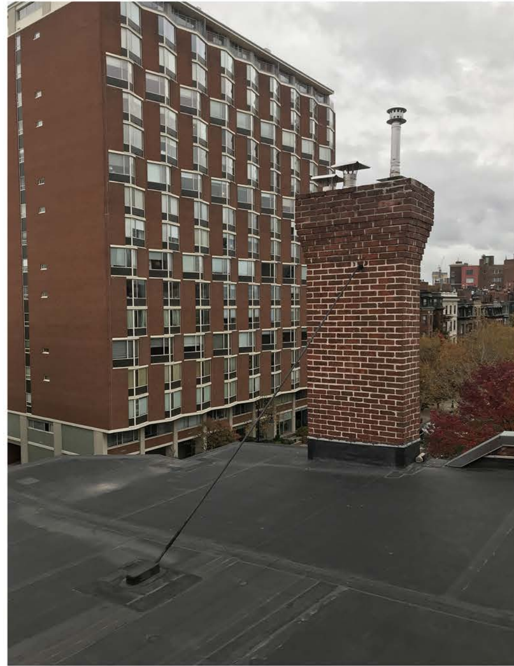
EXISTING FRONT ROOF
