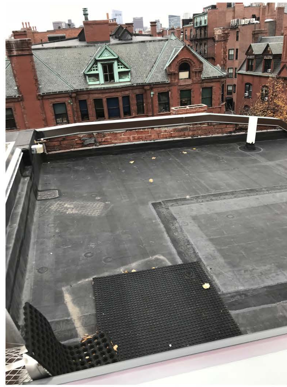
EXISTING REAR ROOF
