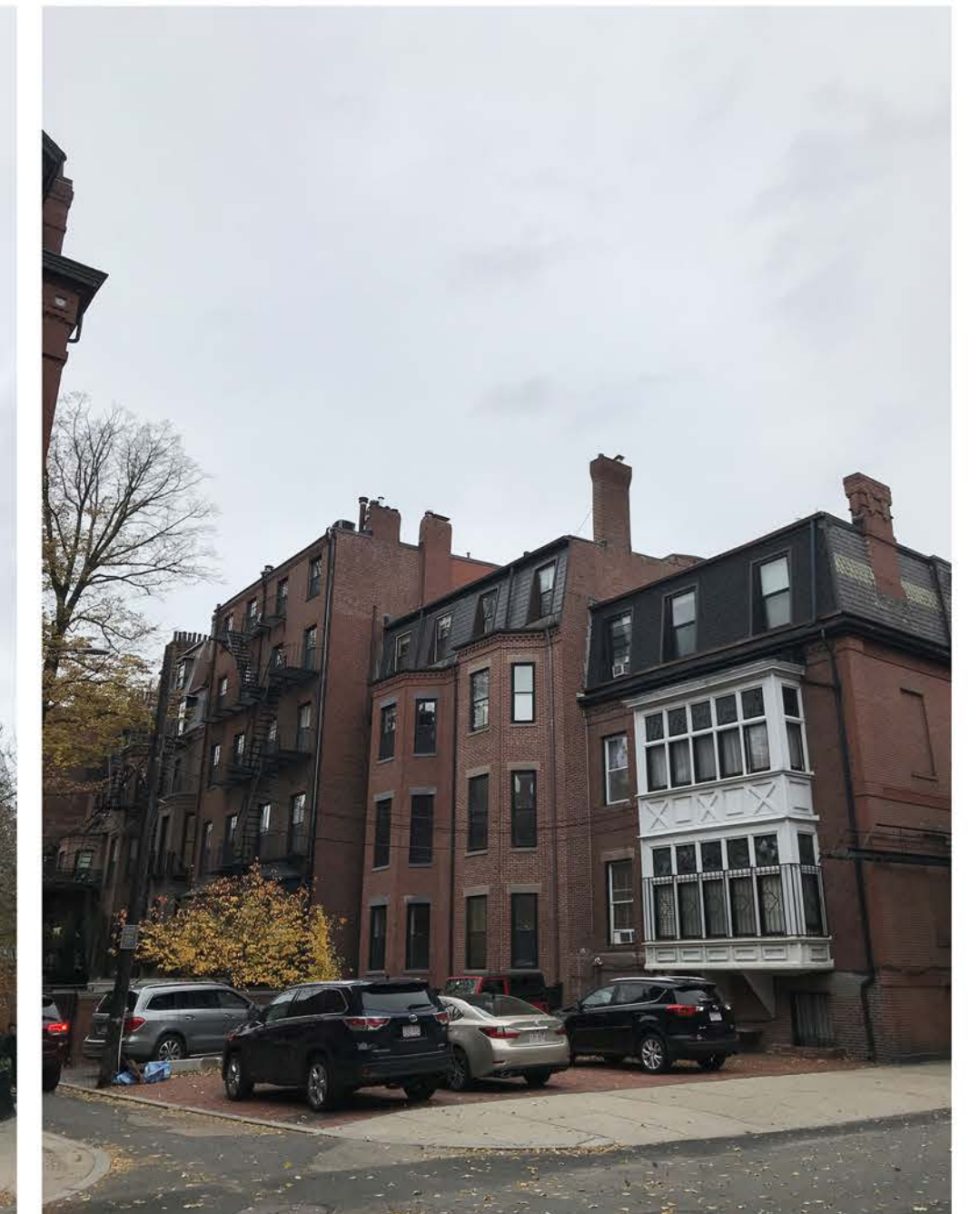
VIEW FROM FAIRFIELD STREET - REAR
