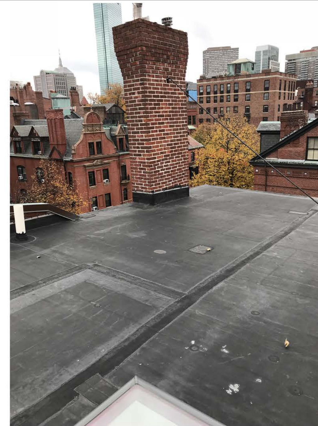
EXISTING REAR ROOF
