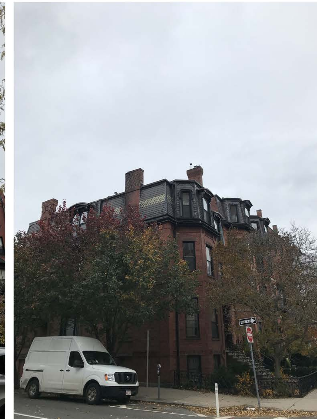
VIEW FROM CORNER OF BEACON STREET AND FAIRFIELD STREET - SIDE
