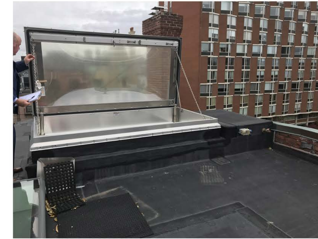
EXISTING ROOF HATCH
