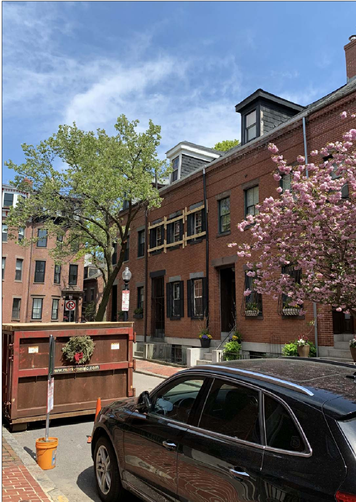
1 EXISTING VIEW 2 - VISIBLE FROM WEST (BOND STREET TOWARD HANSON STREET)
