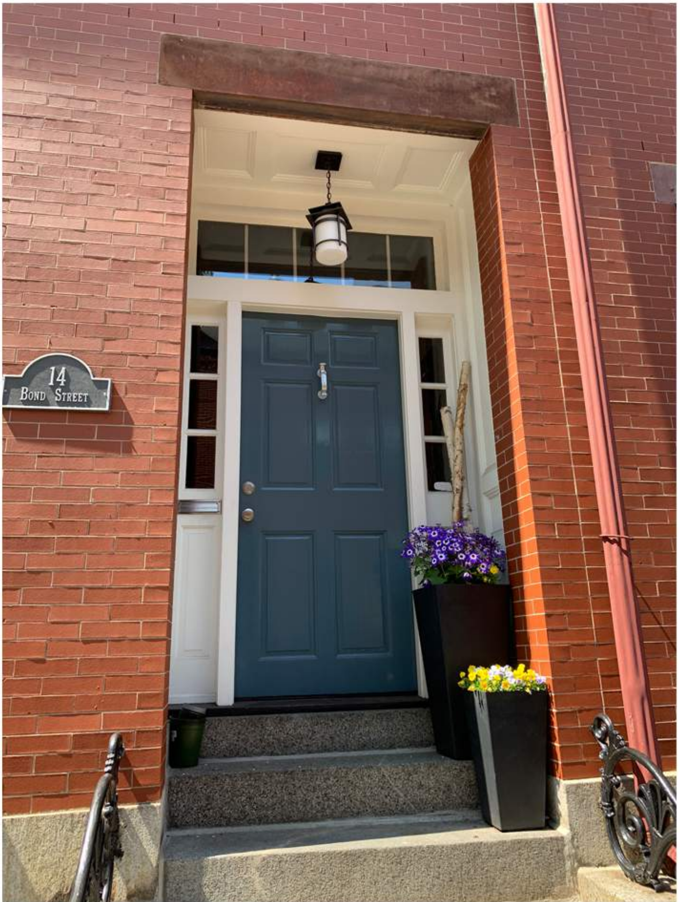
EXISTING ENTRY CONDITIONS AT 14 BOND STREET
