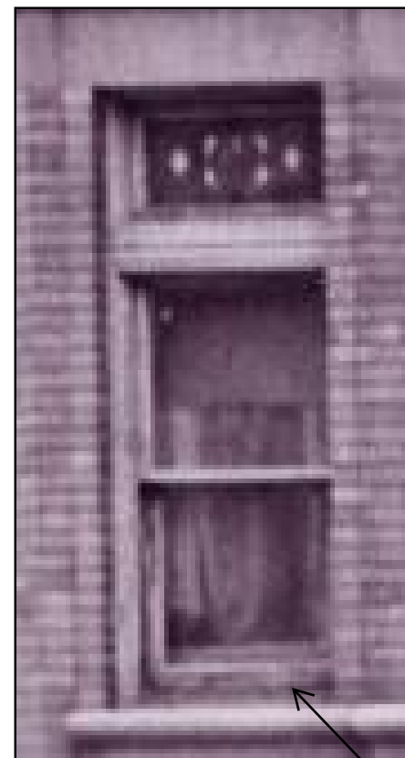
DETAIL C - EXISTING WINDOW BRICK MOLD AT JAMB / SILL
