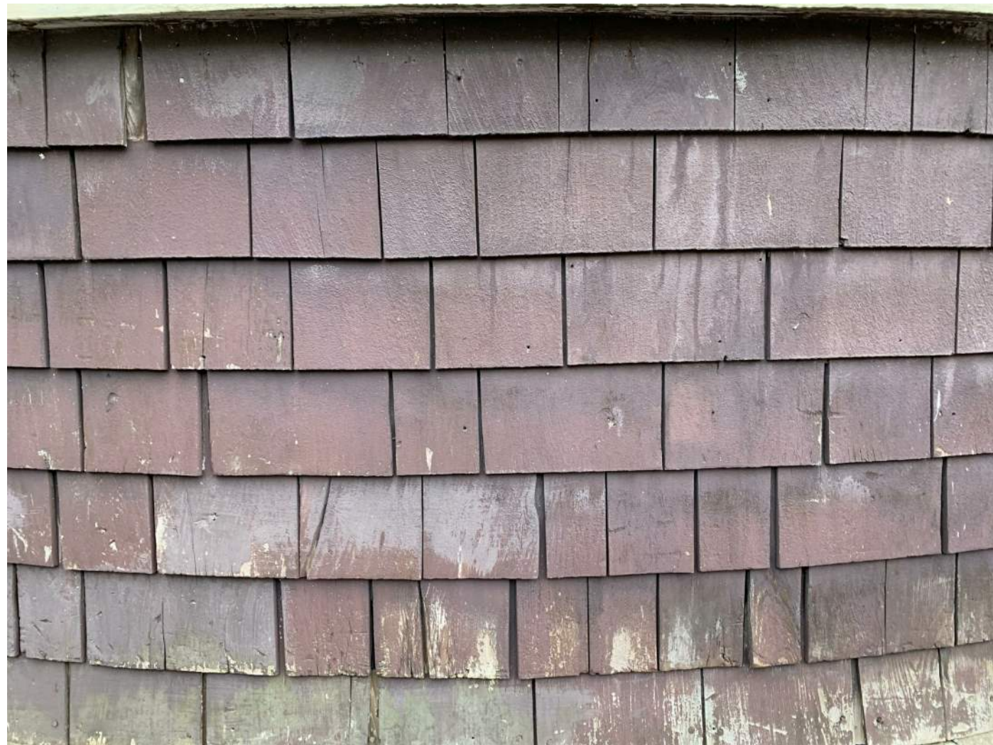
REPAIR AND RESTORE EXISTING SHINGLES. MATCH SIZE AND VARIETY OF EXISTING SHINGLES AT NEW ADDITION FACADES
