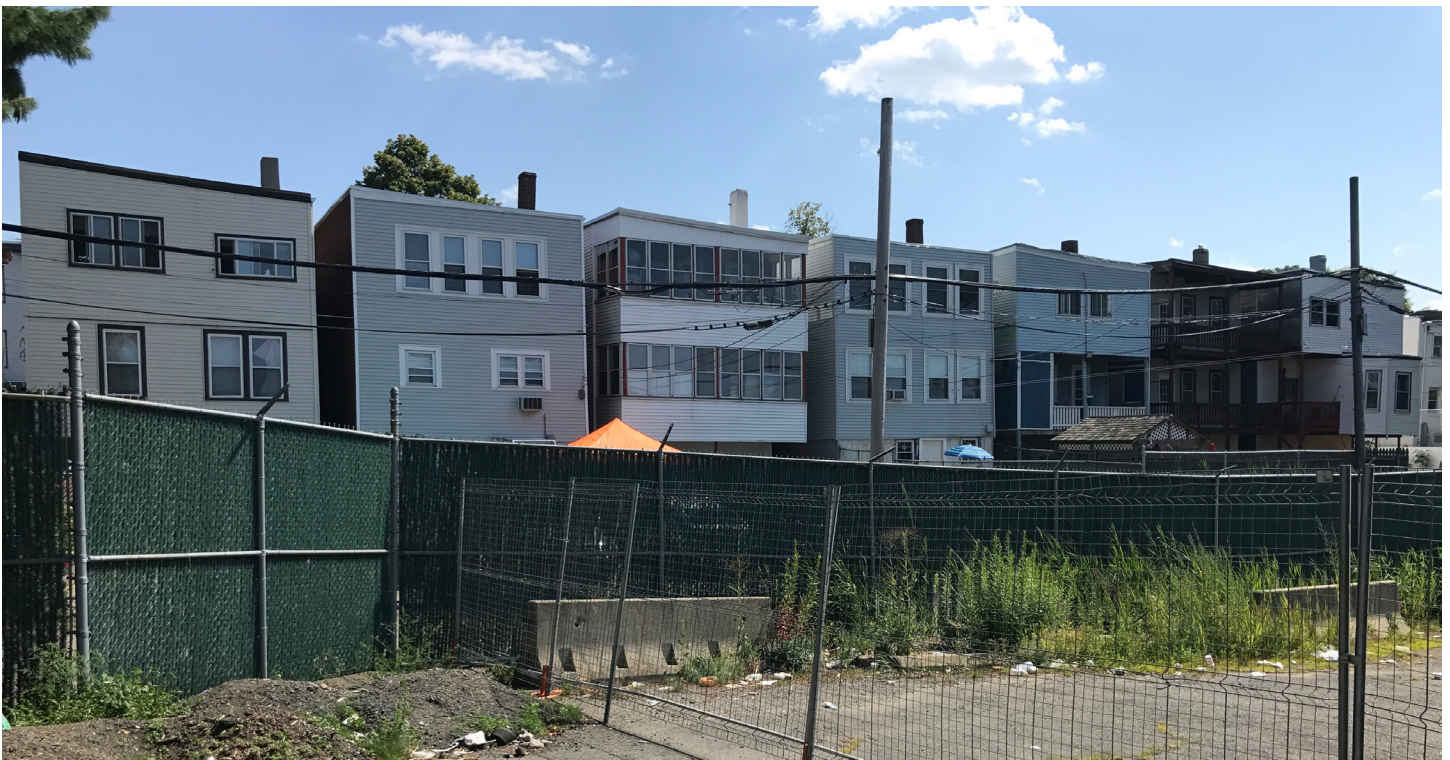
View 4: Eastern edge of Project Site and adjacent rear yards of Saratoga Street homes
