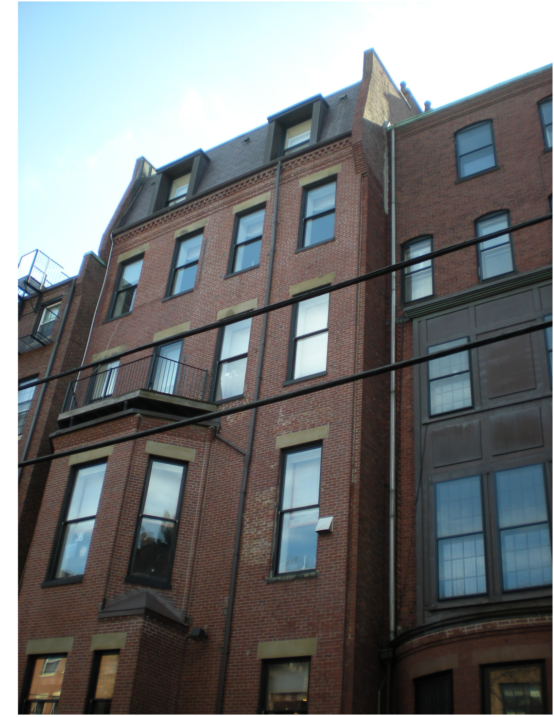
REAR FACADE DETAIL 2018
