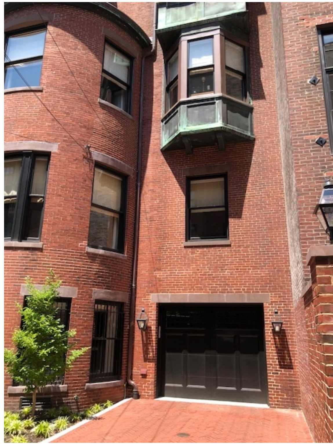
PRECEDENT – GARAGE DOOR IN ORIGINAL FACADE
