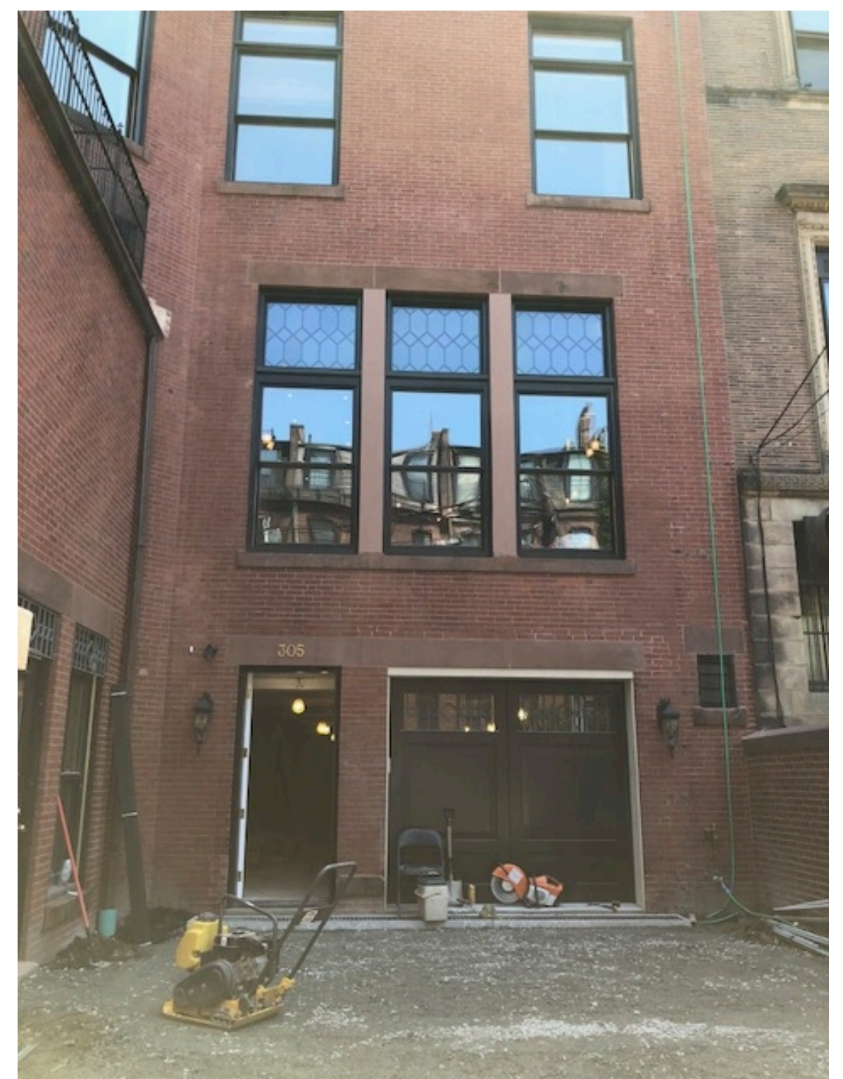
PRECEDENT – GARAGE DOOR IN ORIGINAL FACADE
