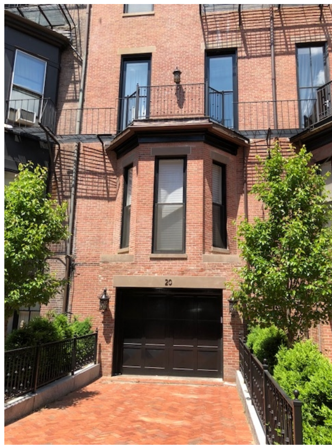
PRECEDENT – GARAGE DOOR IN ORIGINAL FACADE
