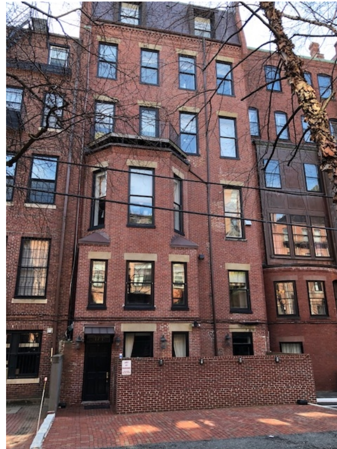
REAR FACADE DETAIL 2018
