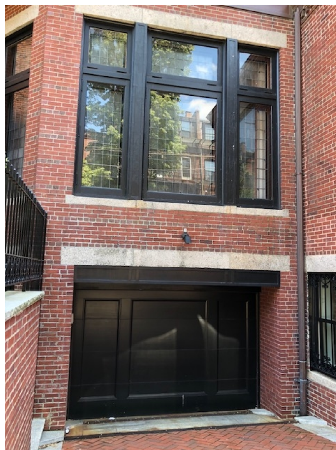
PRECEDENT – GARAGE DOOR IN ORIGINAL FACADE
