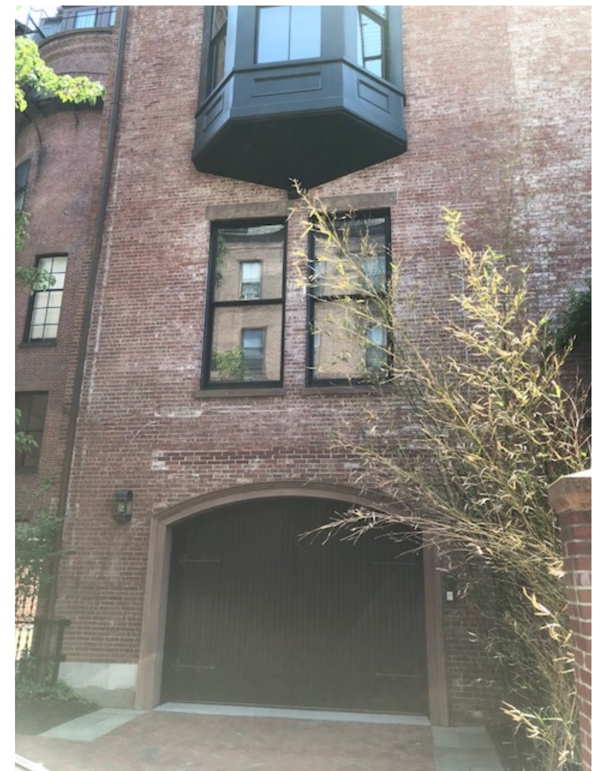
PRECEDENT – GARAGE DOOR IN ORIGINAL FACADE
