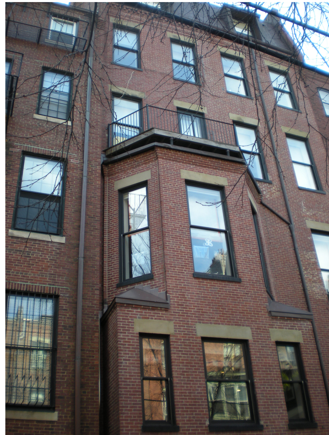
REAR FACADE DETAIL 2018
