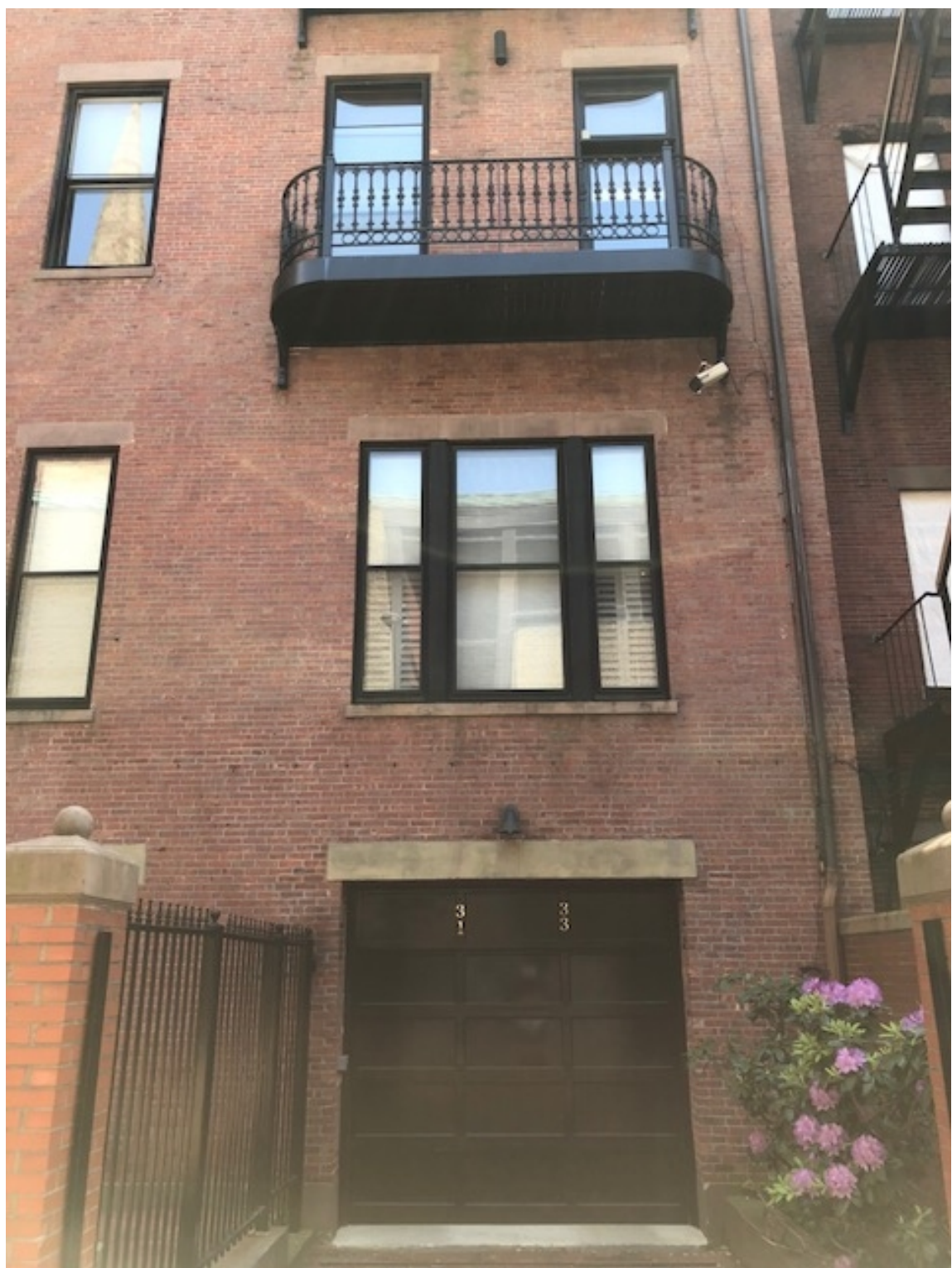
PRECEDENT – GARAGE DOOR IN ORIGINAL FACADE
