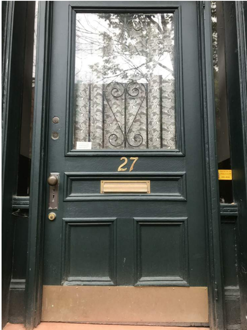
EXISTING FRONT DOOR
