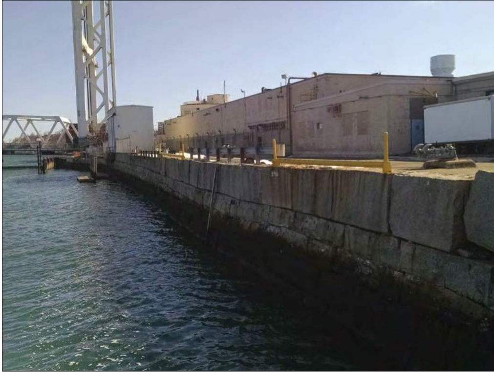
Photograph 1 – East section of existing seawall visible above waterline.
