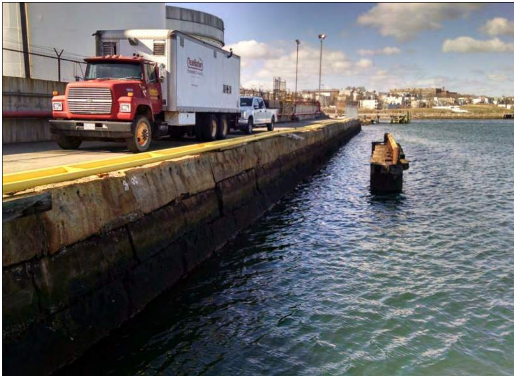
Photograph 2 – West section of existing seawall visible above waterline.
