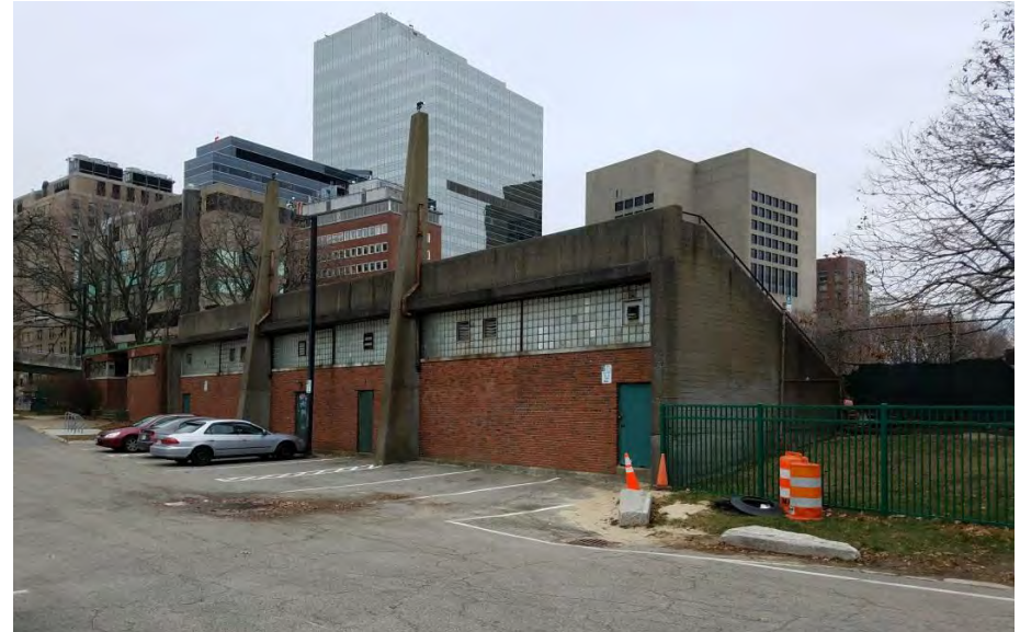
2. View looking southeast to side of Building
