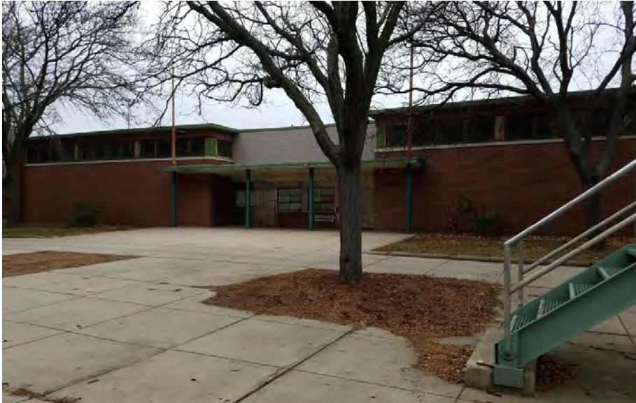
1. View looking west to front of building
