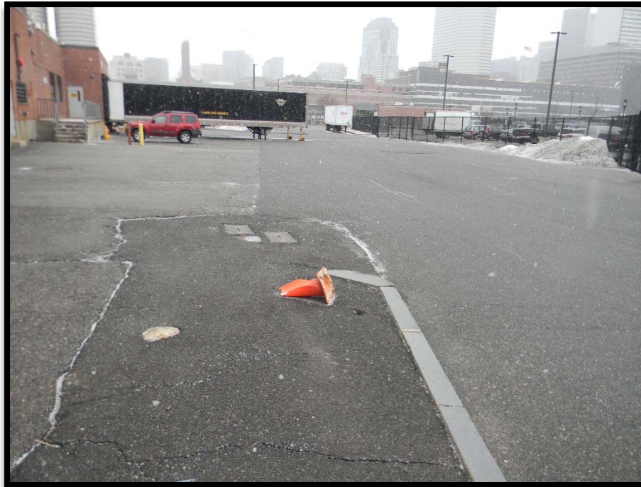
Photo 07 – Looking west at Driveway
