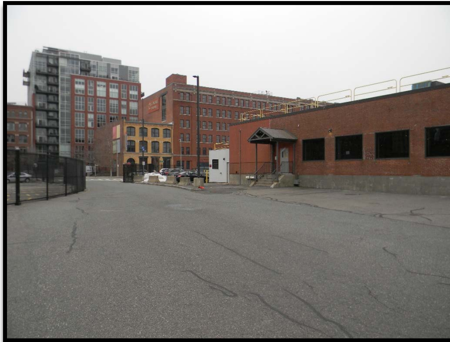
Photo 05 – Looking southeast at Project location
