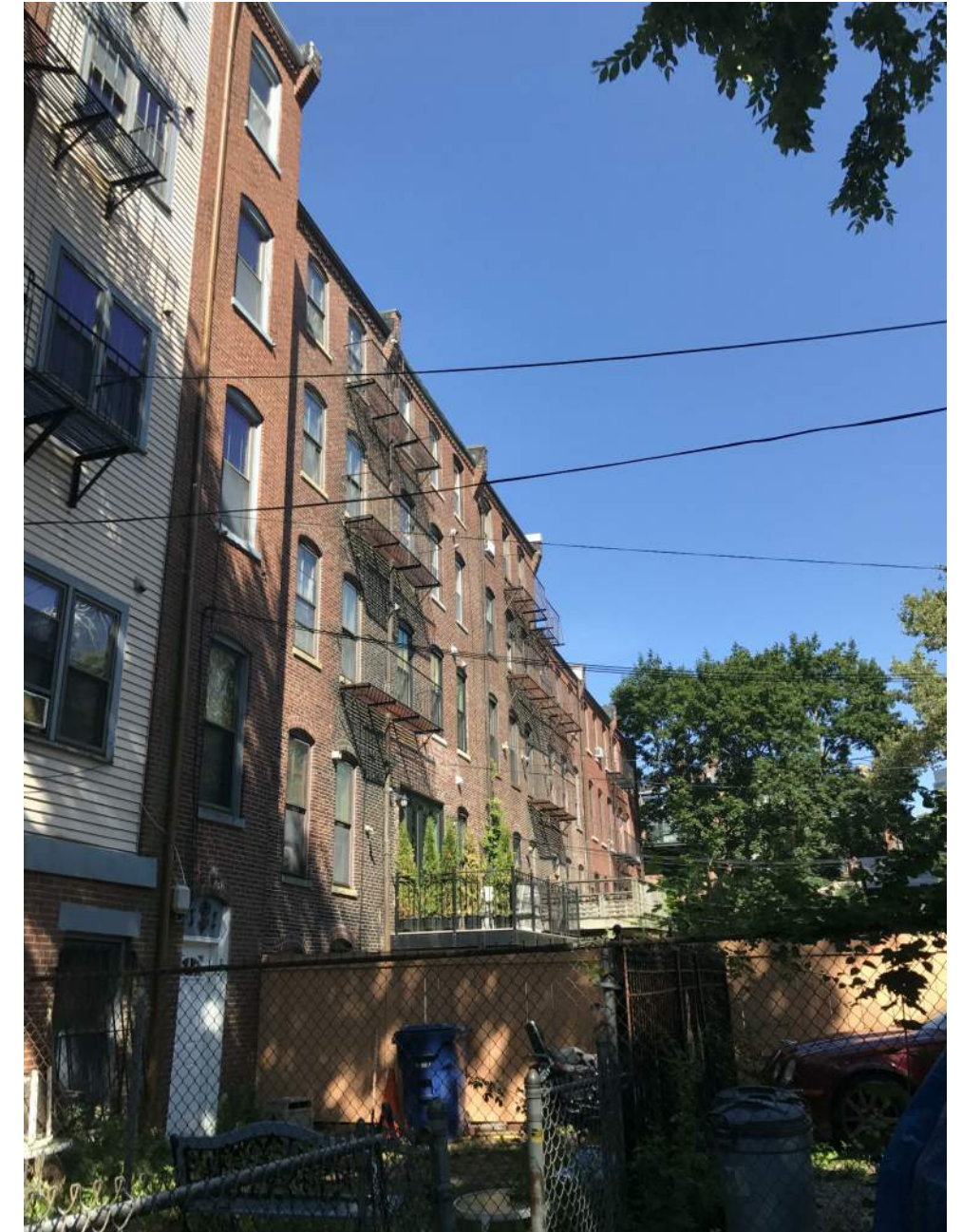
REAR ALLEY FACING NORTH
